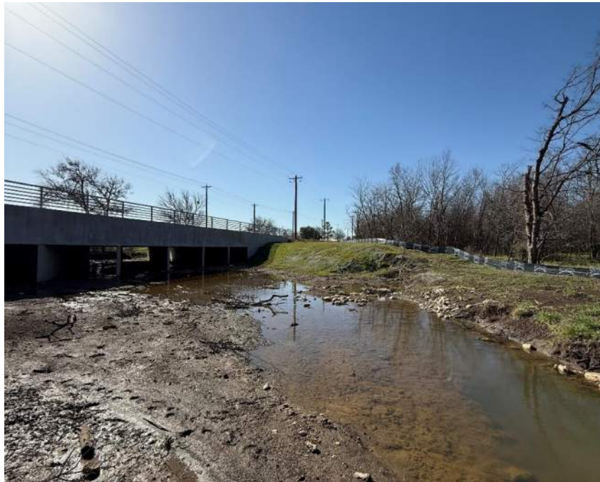
Photo 17: Discharge Point 2 Transect 2, Downstream
