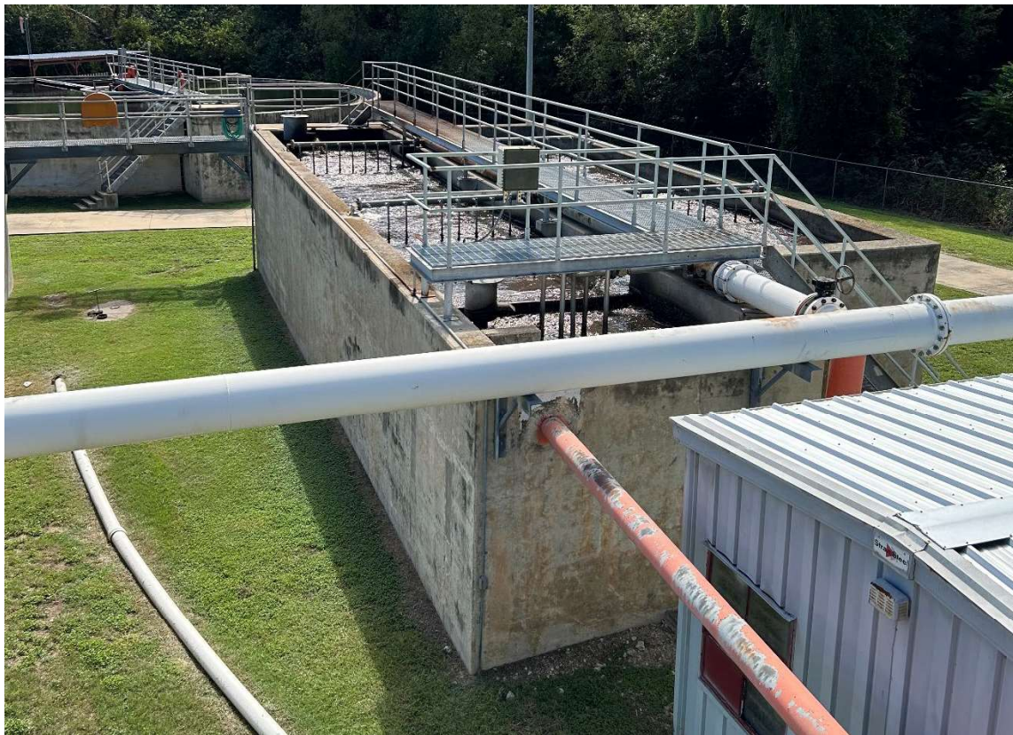
Sludge Digester
