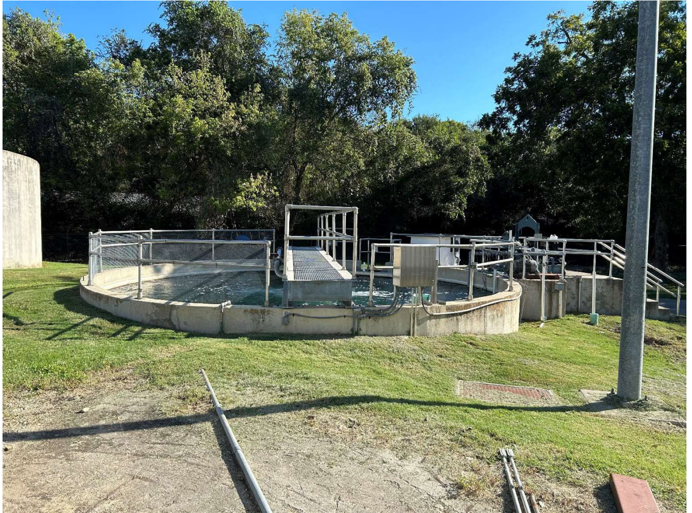
Chlorine Contact Chamber
