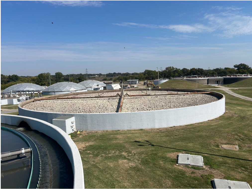
Photograph 5. Trickling Filter 1
