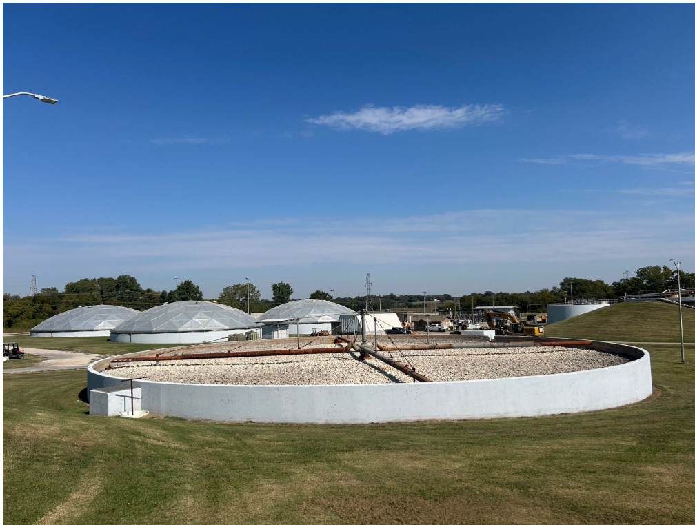
Photograph 6. – Trickling Filter 2
