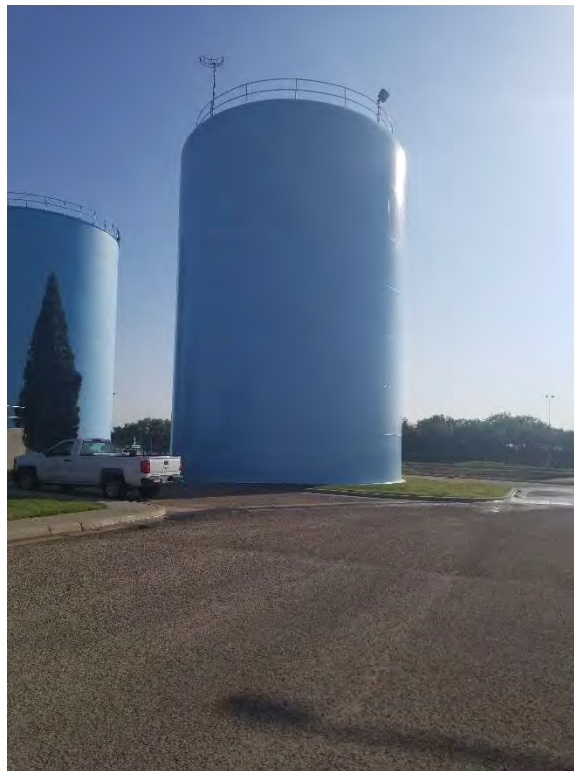
South Backwash Tank, 1965
