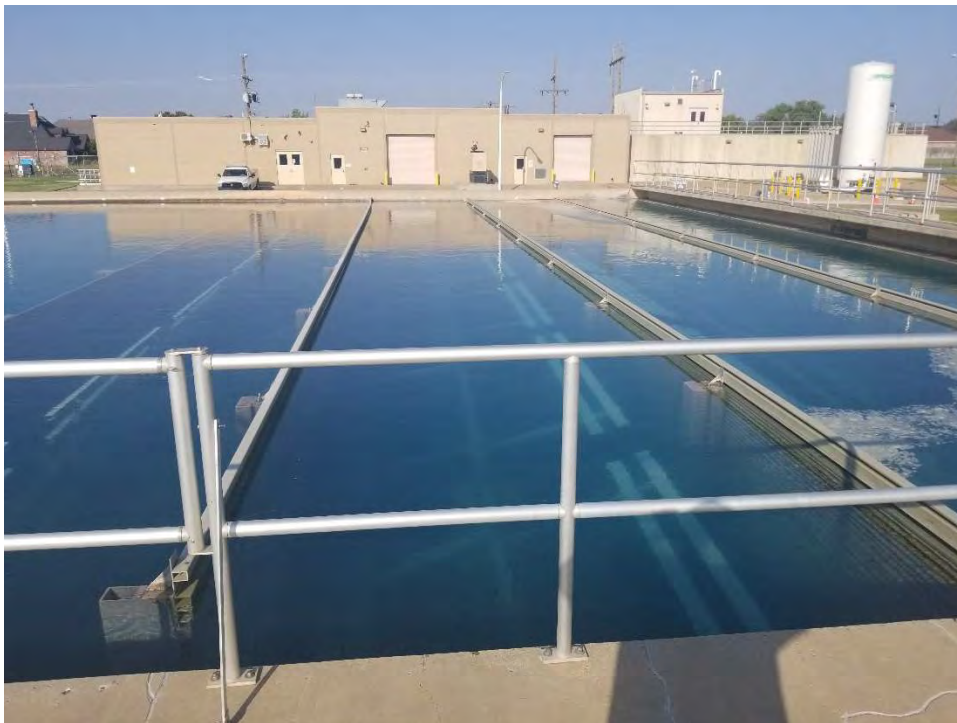
West Flocculator Basin, 1965
