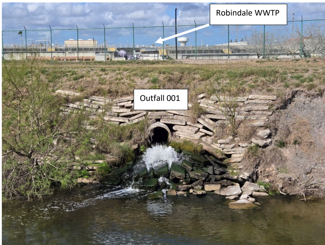
Robindale Wastewater Treatment Plant Outfall 001 – Existing effluent disposal site.
