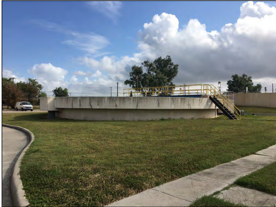
Photograph 1: Photograph of Primary Clarifier 1
