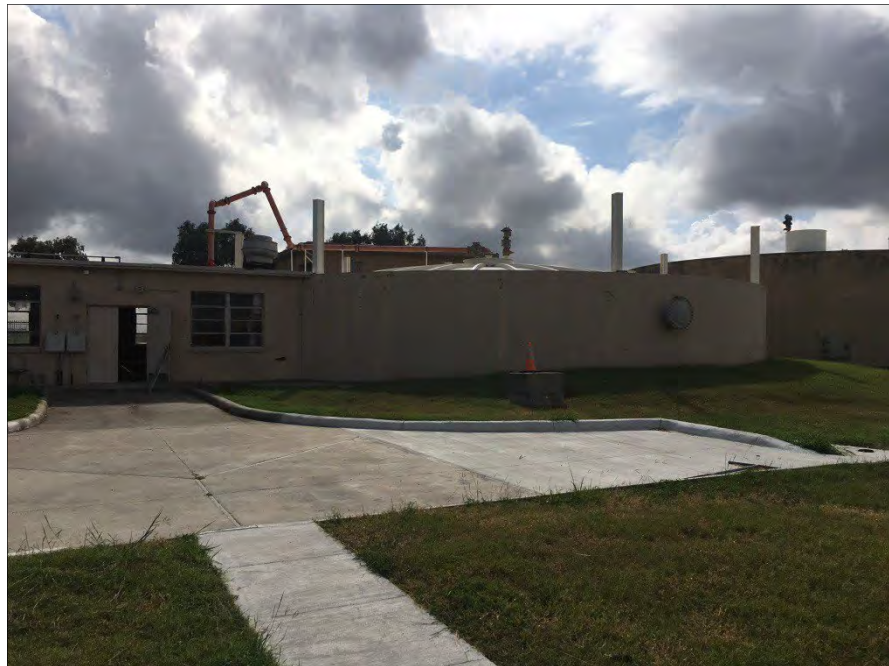
Photograph 6: Photograph of Sludge Digester 2.
