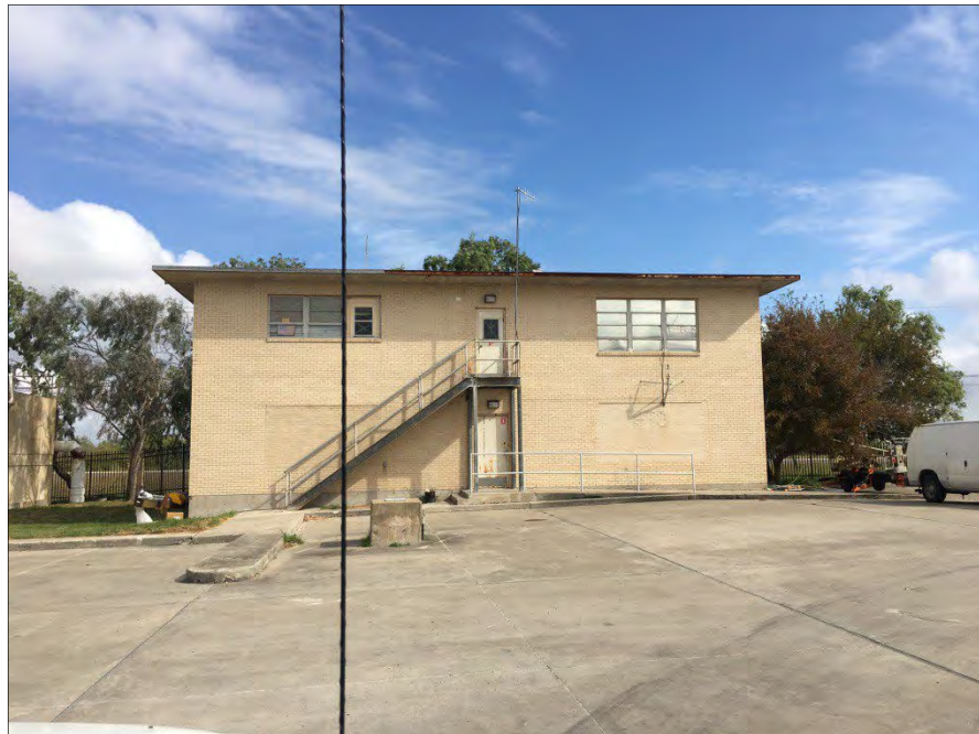
Photograph 4: Photograph of Electrician Building.
