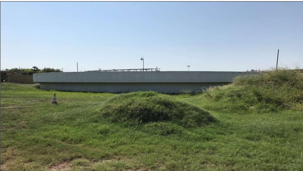
Photograph 2: Photograph of Decommissioned Trickling Filter No. 6
