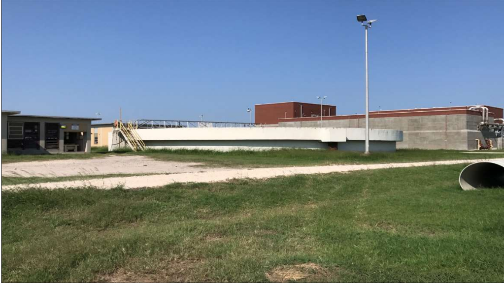
Photograph 23: Photograph of Decommissioned Primary Clarifier No. 2
