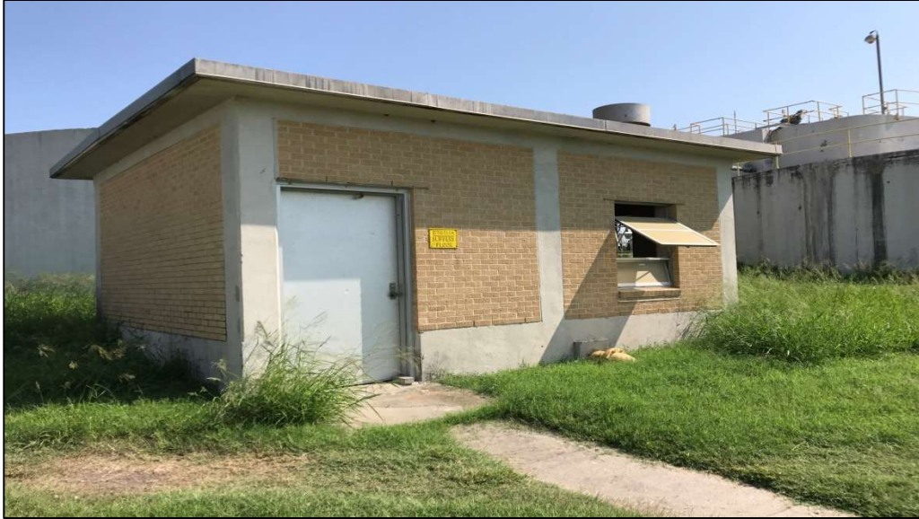
Photograph 3: Photograph of the Decommissioned Pump Building
