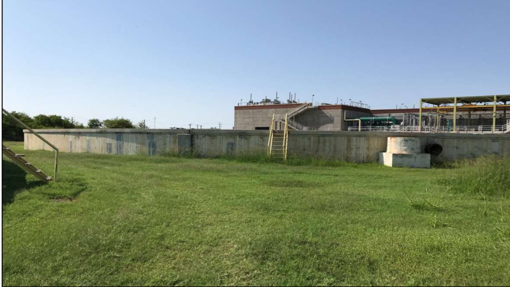
Photograph 11: Photograph of Decommissioned Trickling Filter No. 1
