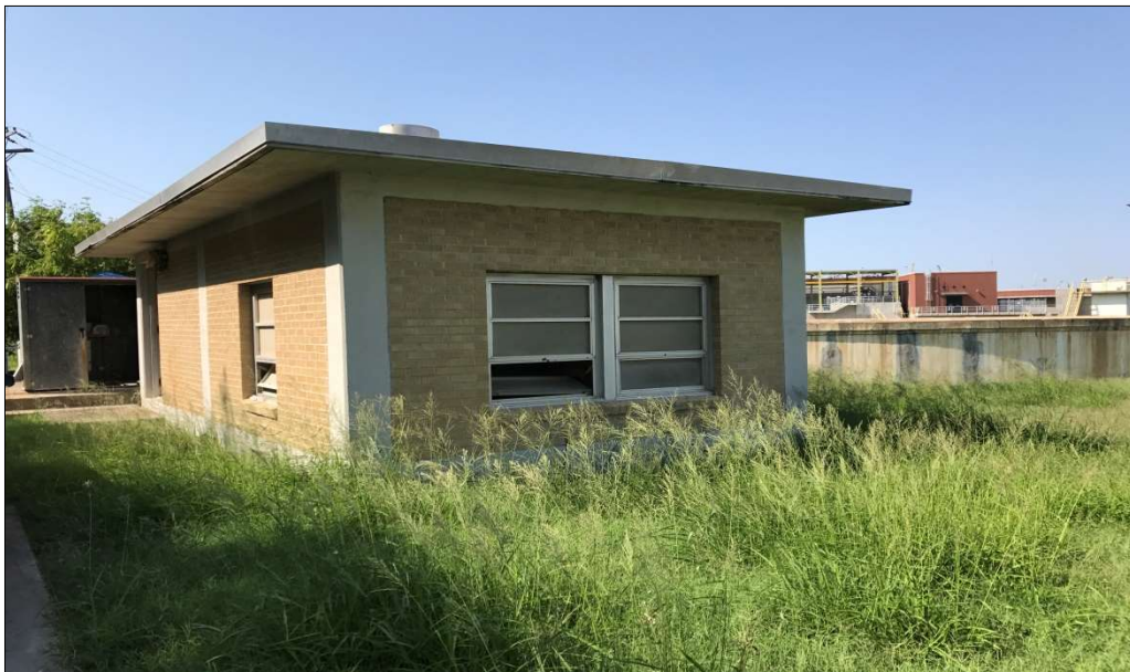
Photograph 4: Photograph of the Decommissioned Stand-by Generator Building
