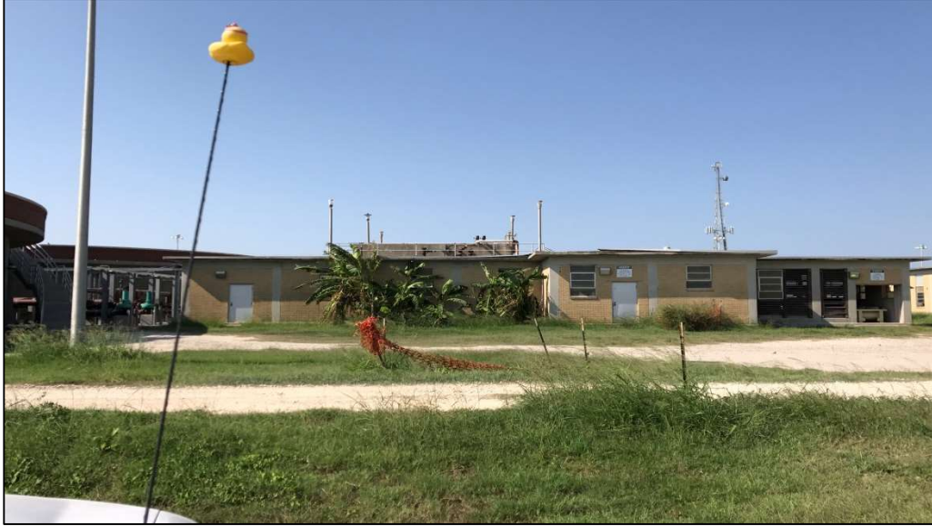
Photograph 25: Photograph of Decommissioned Blower Building
