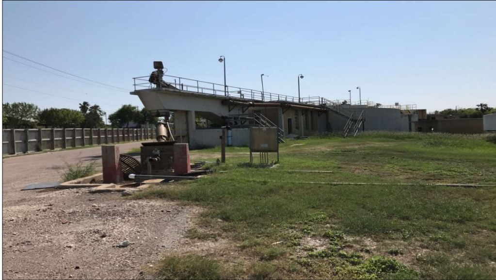
Photograph 7: Photograph of the Decommissioned Grit Removal and Decommissioned Return Flow Re-conditioner (RFR) Building
