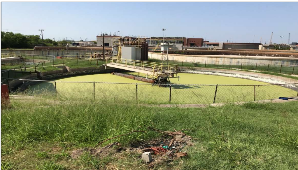
Photograph 16: Photograph of Decommissioned Final Clarifier No. 2
