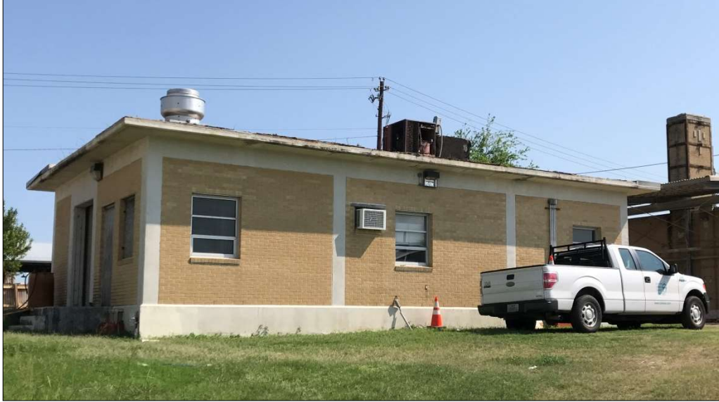
Photograph 5: Photograph of the Decommissioned Main Pump House
