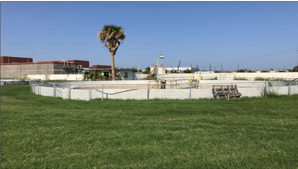
Photograph 20: Photograph of Decommissioned Intermediate Clarifier No. 2
