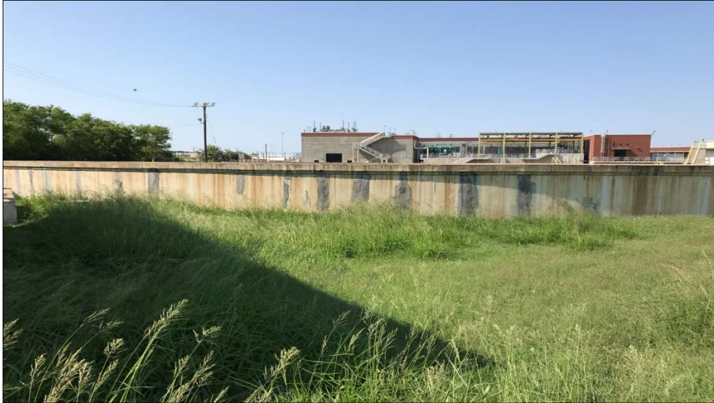
Photograph 13: Photograph of Decommissioned Trickling Filter No. 3
