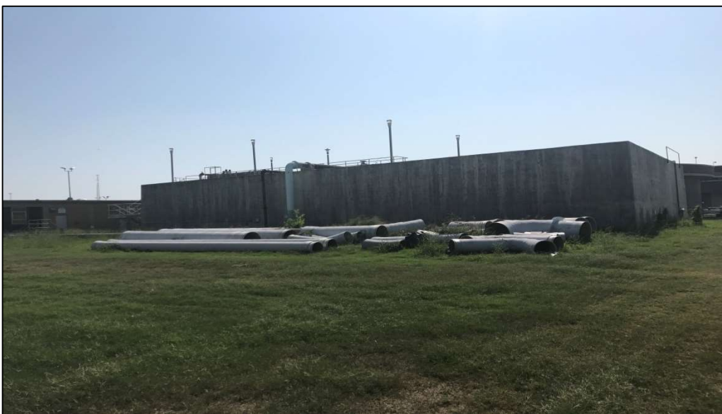
Photograph 10: Photograph of the Decommissioned Digesters
