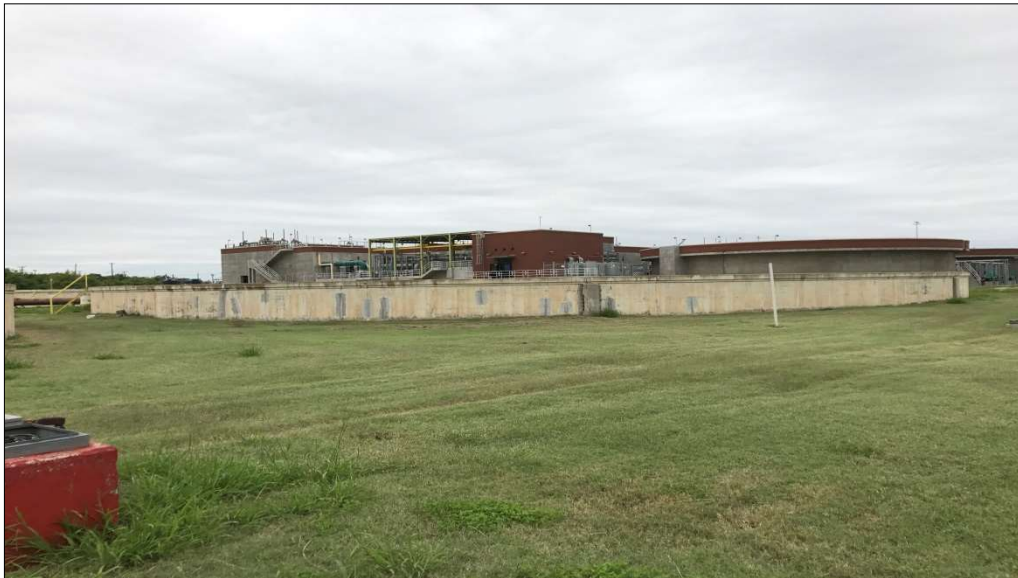
Photograph 12: Photograph of Decommissioned Trickling Filter No. 2
