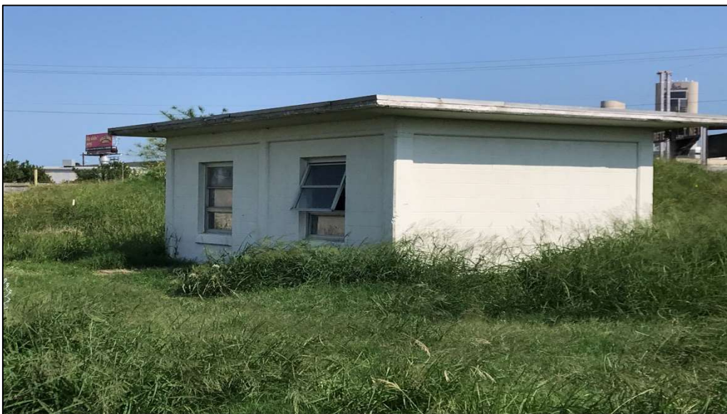
Photograph 18: Photograph of Decommissioned Pump Building
