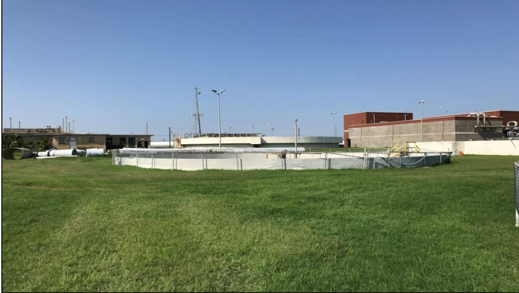
Photograph 19: Photograph of Decommissioned Intermediate Clarifier No. 1
