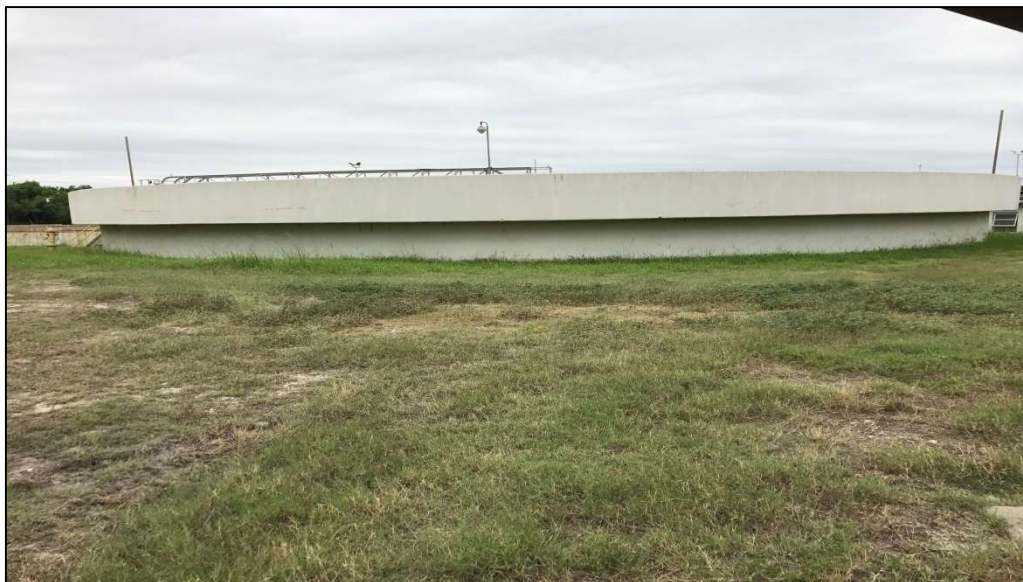
Photograph 24: Photograph of Decommissioned Primary Clarifier No. 1
