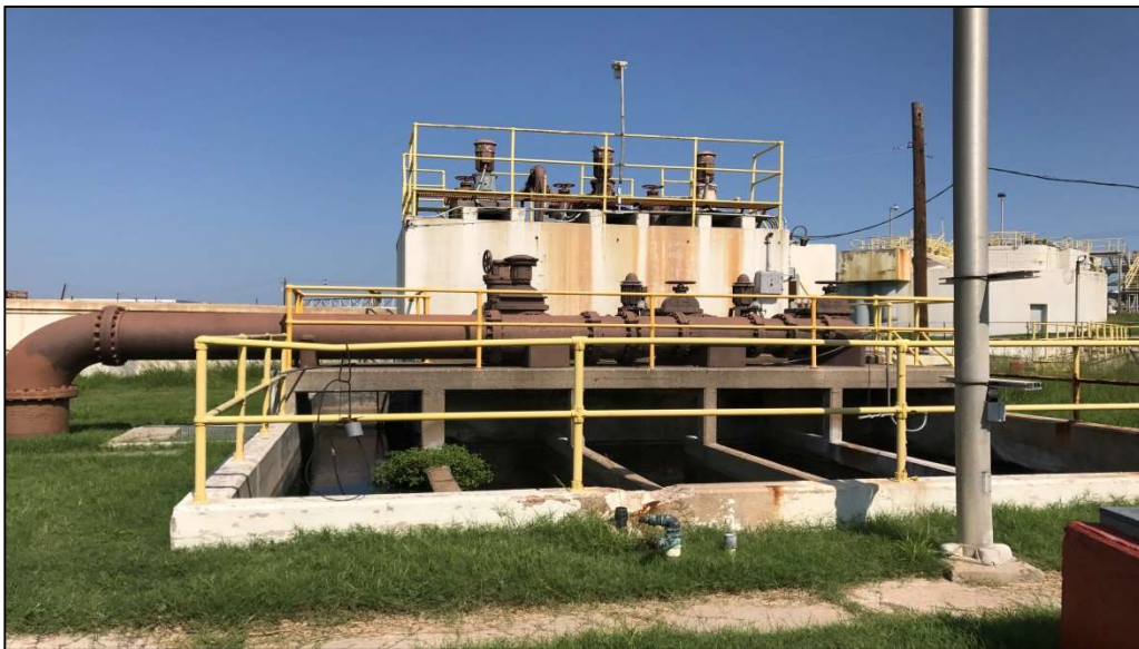
Photograph 8: Photograph of the Decommissioned Chlorine Contact Chamber
