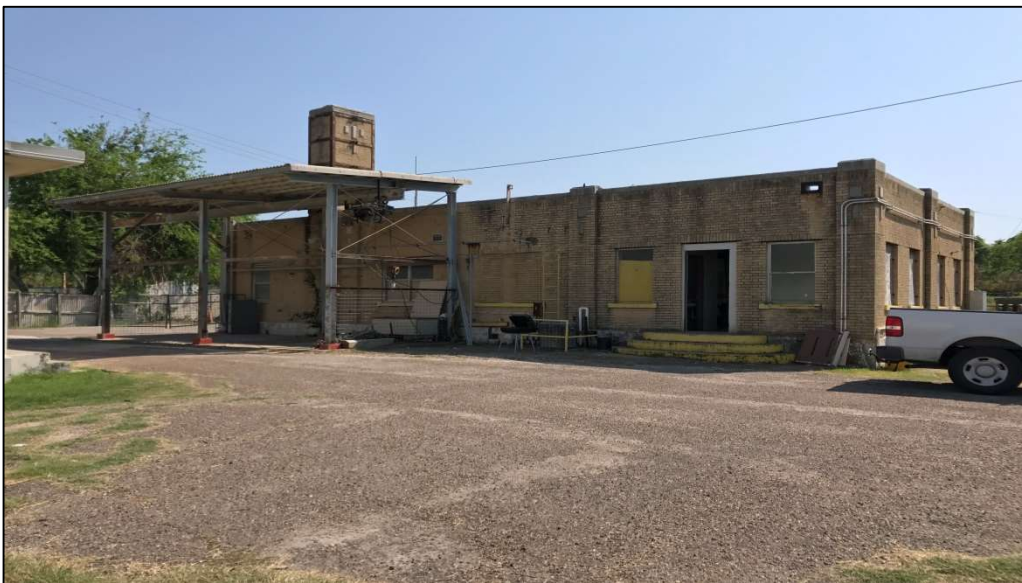
Photograph 22: Photograph of the Original Office Building
