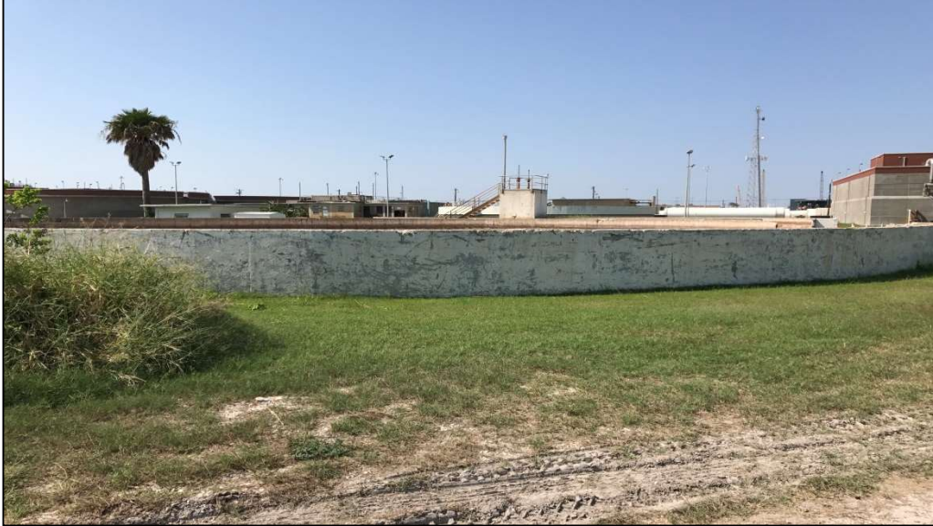
Photograph 1: Photograph of Decommissioned Trickling Filter No. 5
