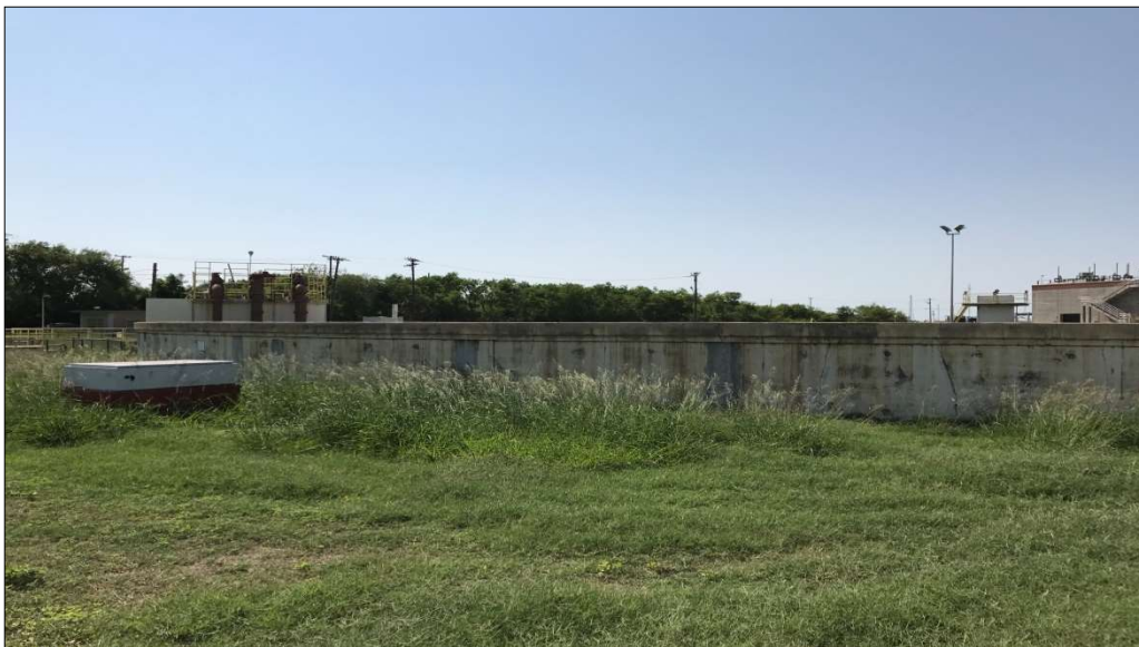
Photograph 14: Photograph of Decommissioned Trickling Filter No. 4
