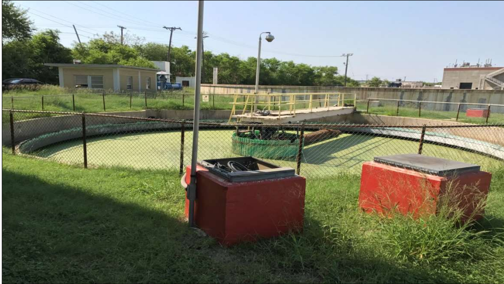
Photograph 15: Photograph of Decommissioned Final Clarifier No. 1
