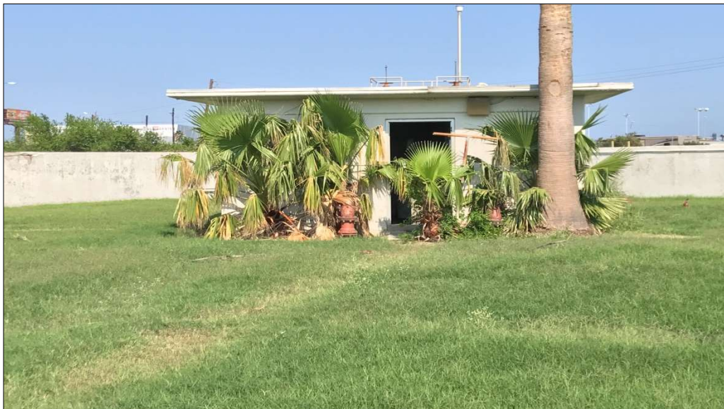
Photograph 26: Photograph of Decommissioned Pump House
