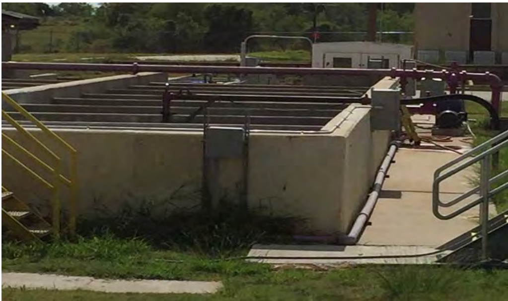
Photograph 4: Chlorine contact basins
