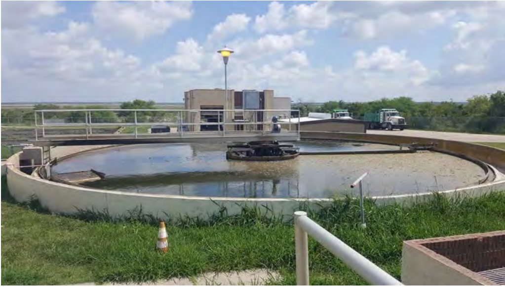
Photograph 1: Post-thickener
