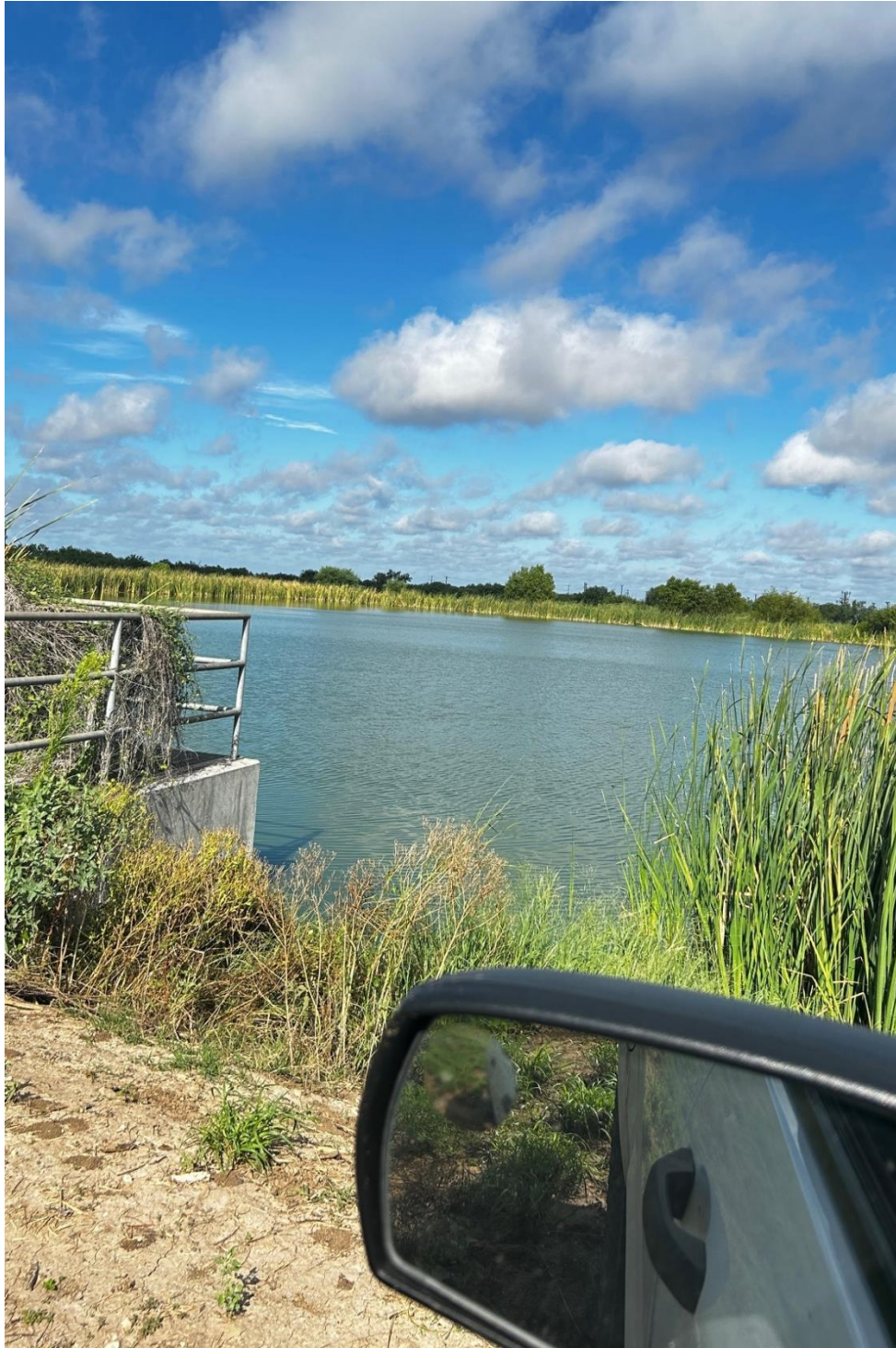
Photograph 1 – Existing treatment pond (to be decommissioned).
