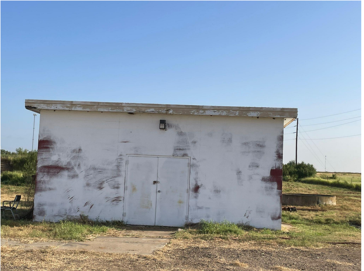
Photograph 5 – Existing prison list station pumps building.
