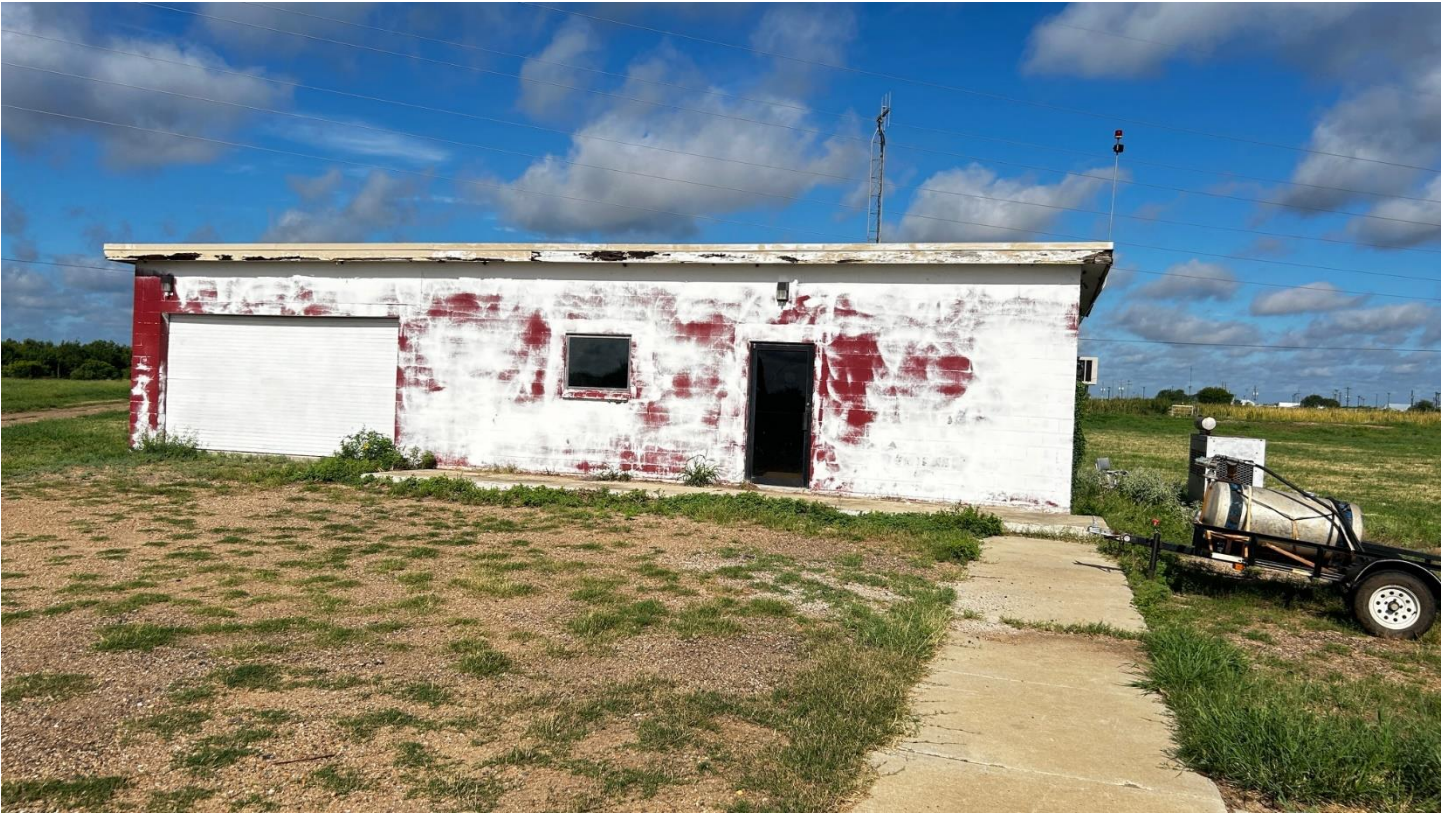
Photograph 4 – Existing prison office.
