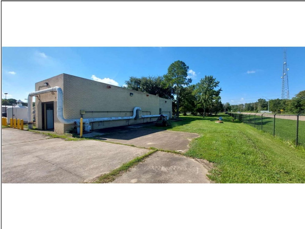
Photo 11 – Main Lift Station Building
