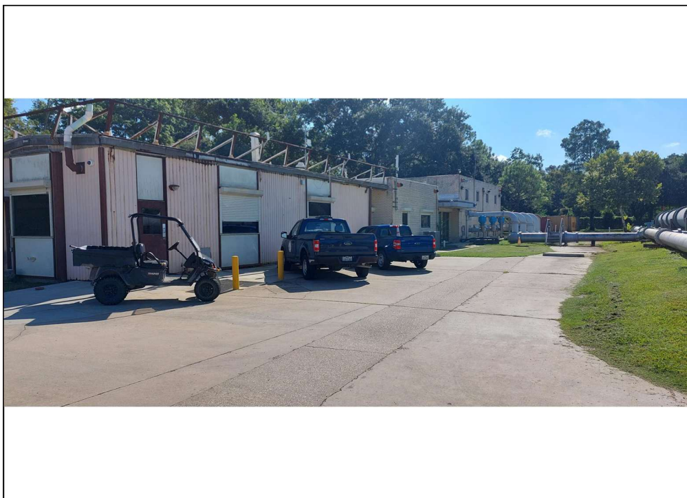
Photo 1 – Administration-Control Room-Blower 1 Building
