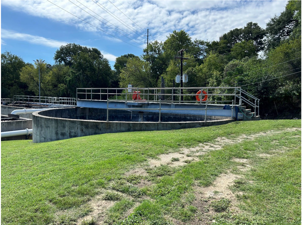
Sludge Thickener
