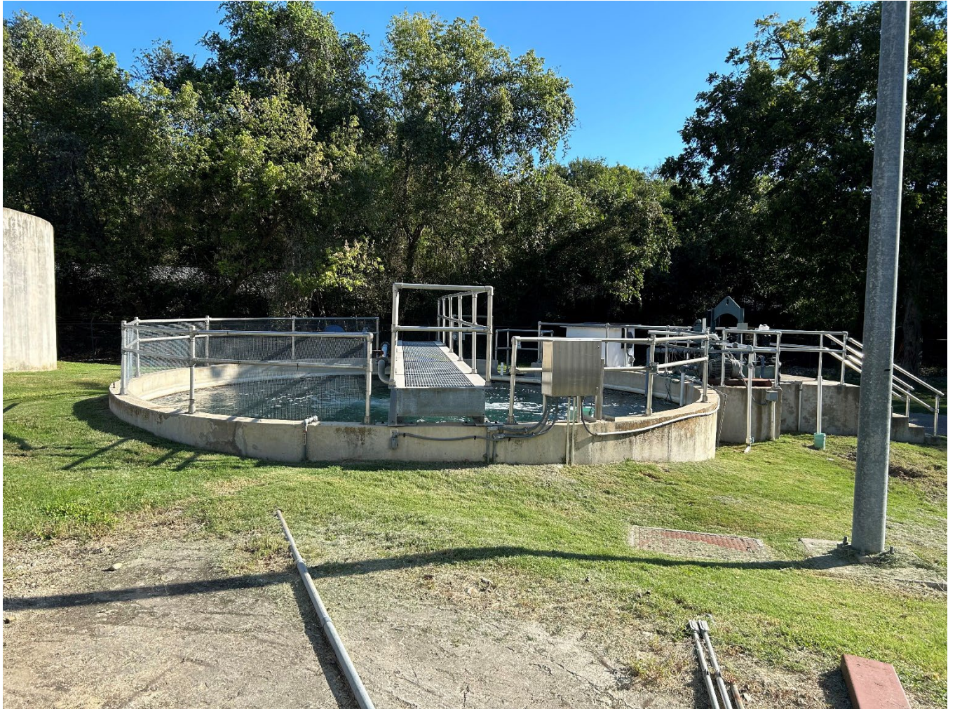
Chlorine Contact Chamber
