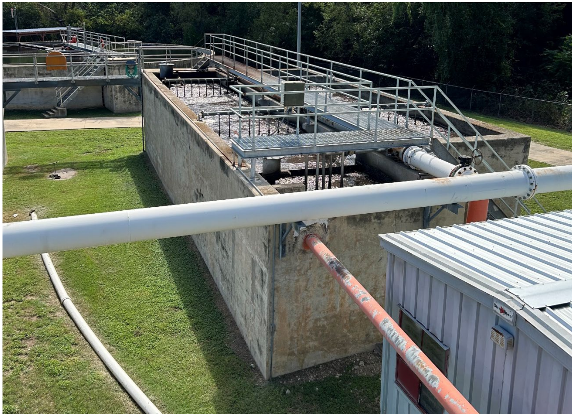
Sludge Digester
