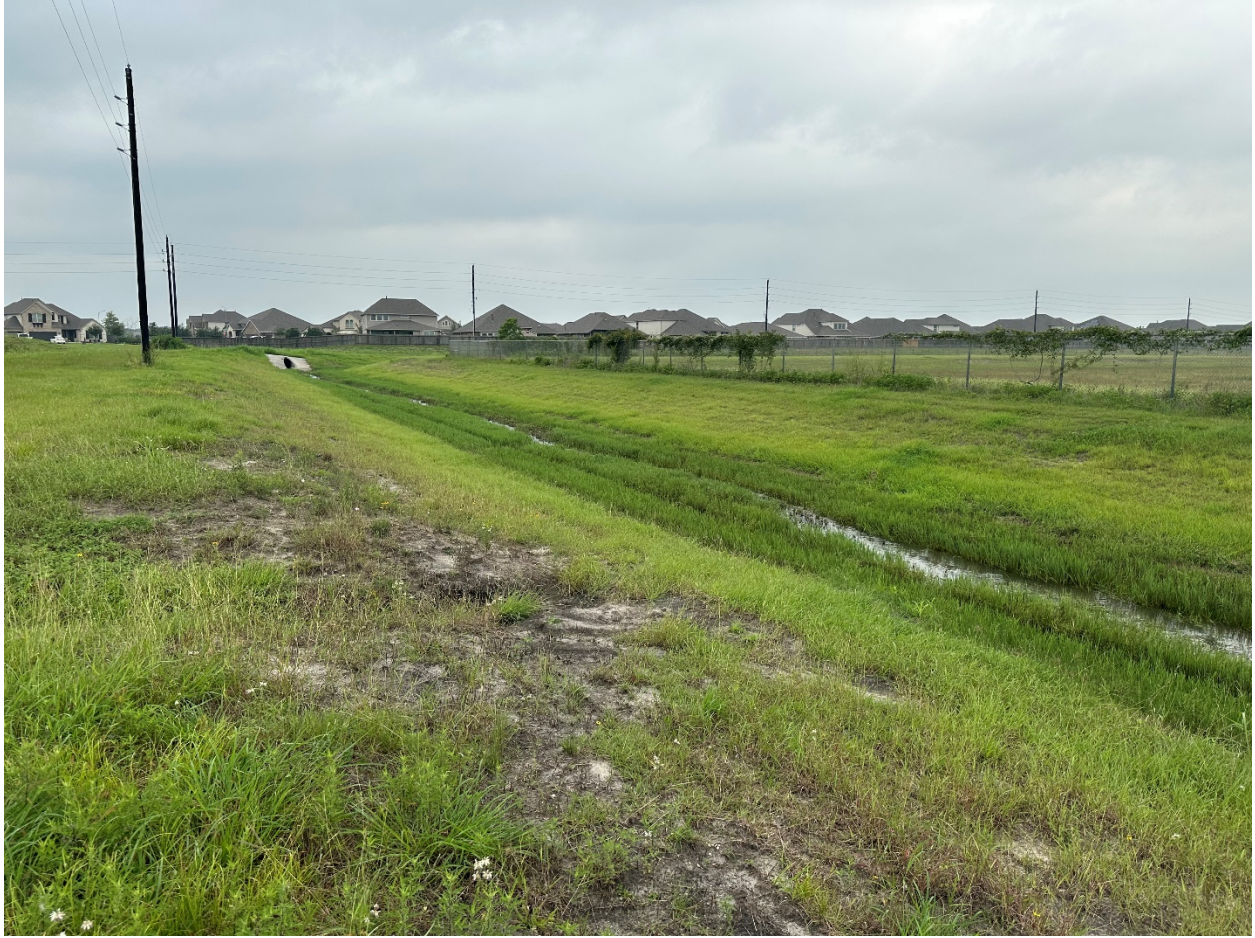
Photo 3. Outfall 002 and Flood Control Drainage Ditch, looking upstream.
