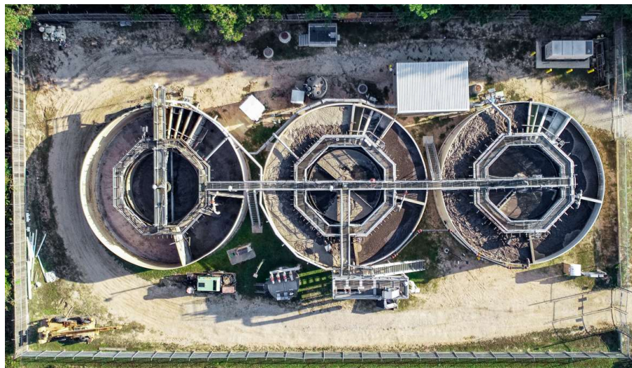
Figure 2: Existing 0.675 MGD WWTP
