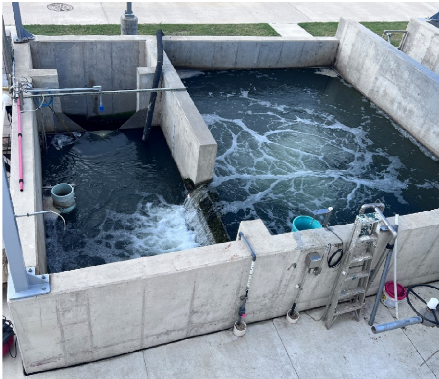
Photo 13: NPW Basin With New Plate Aerators
