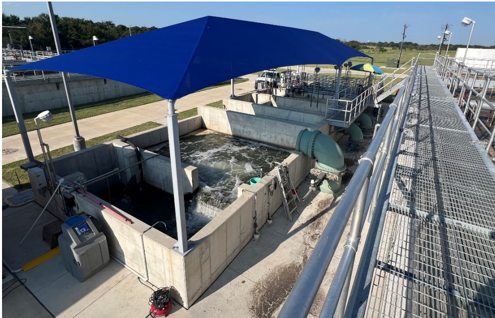
Photo 9.0: Overview of Filter Basins with New Shade Cloth Structure
