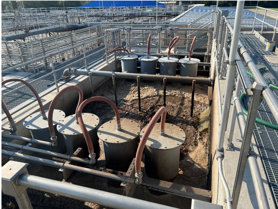
Photo 3.0: 10" Airlift Pumps in Rapid Mix Basin, Looking South
