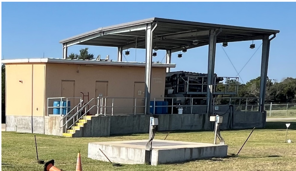
Photo 15.0: Roof Improvements Over Belt Press Facility
