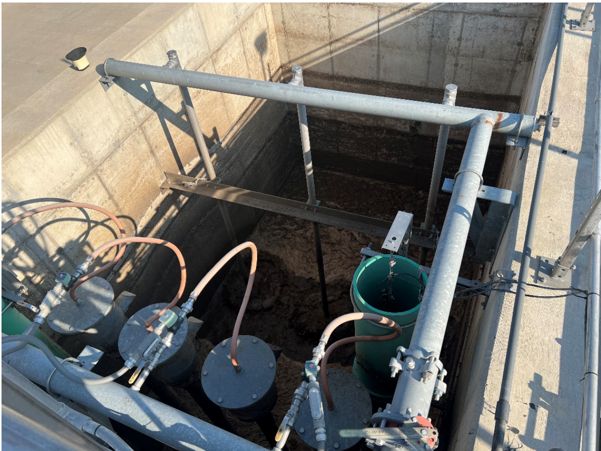
Photo 2.0: Three (3) New - 4" Airlift Pumps in WAS Basin
