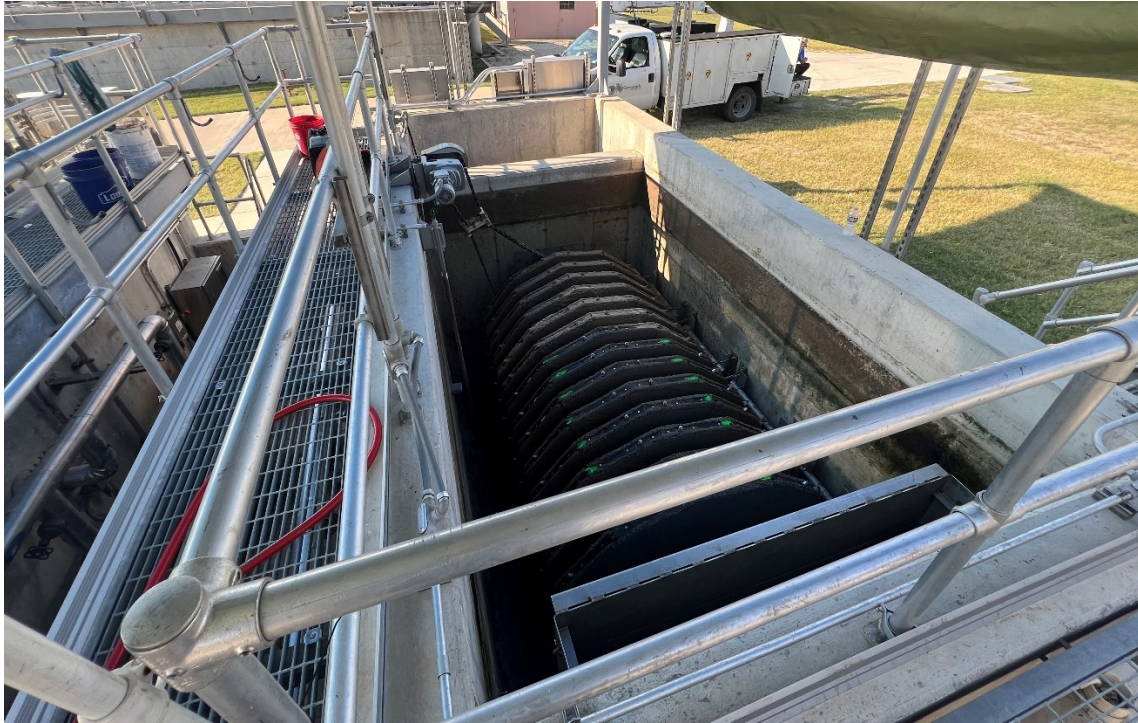
Photo 11.0: Example of Existing Filter Basin 1 Cloth Media Filter (Not an Improvement)
