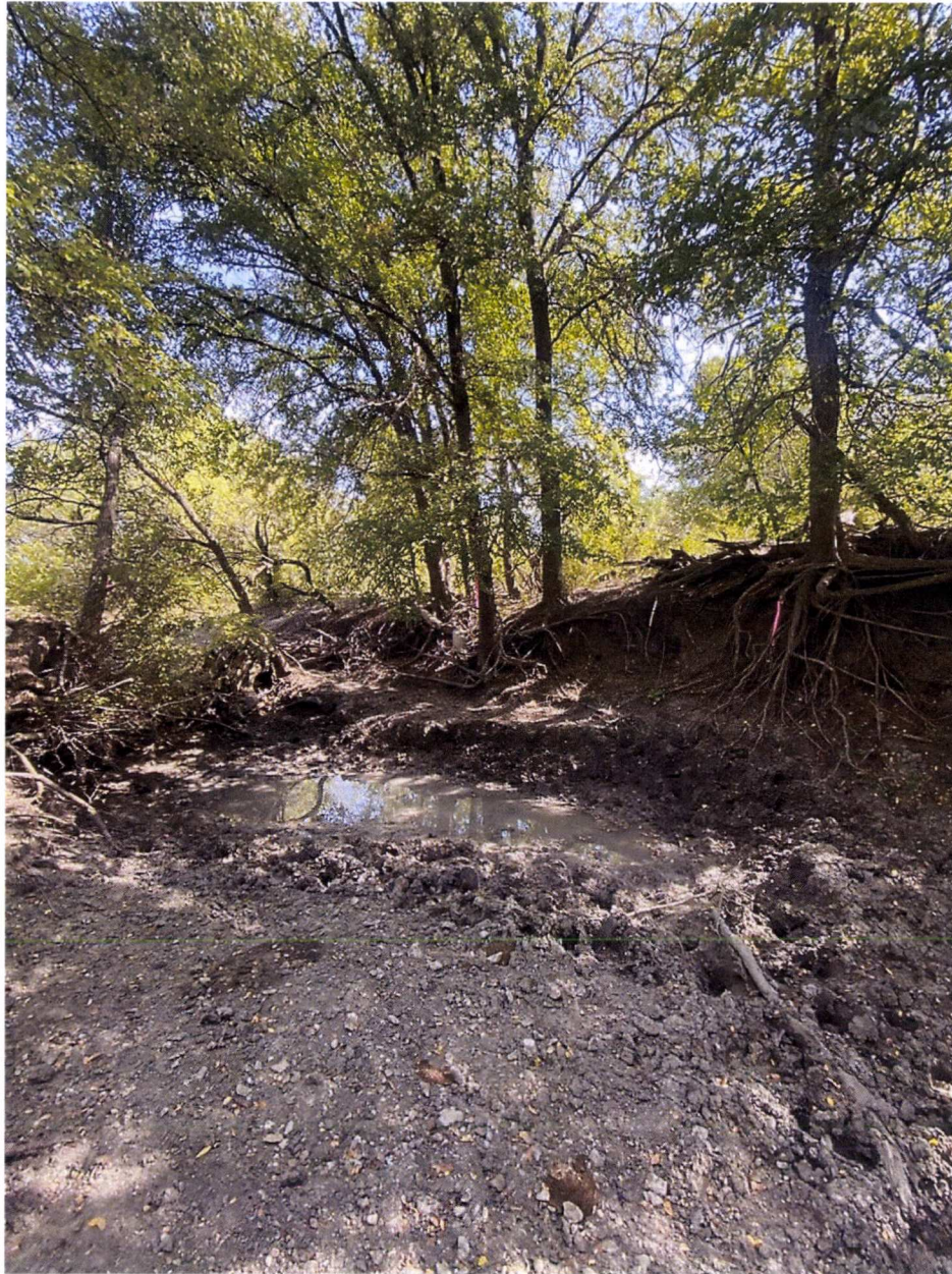
Photo 2: Downstream of discharge point
