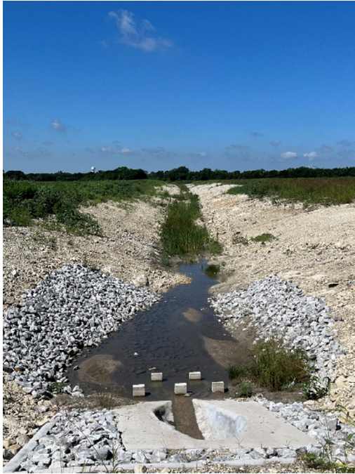
Photo 1: Downstream of discharge location into graded channel
