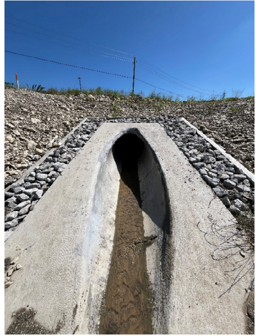
Photo 2: Upstream of discharge location into the concrete storm sewer pipe
