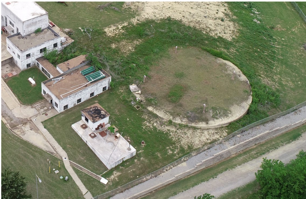
Photograph 4: In-Ground Clearwell and High-Service Pump Station (original) – Originally constructed, ca. 1941 (decommissioned in 1993).
