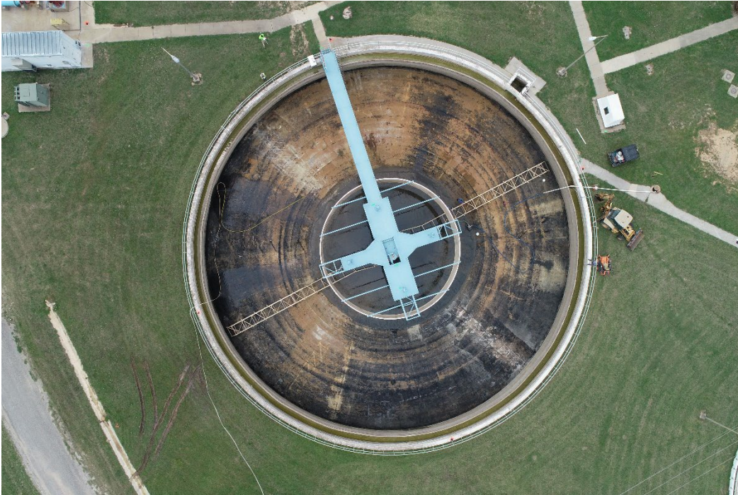
Photograph 1: Clarifier No. 2 – Originally constructed as clariflocculator in 1978; converted to solids contact clarifier in 1993.
