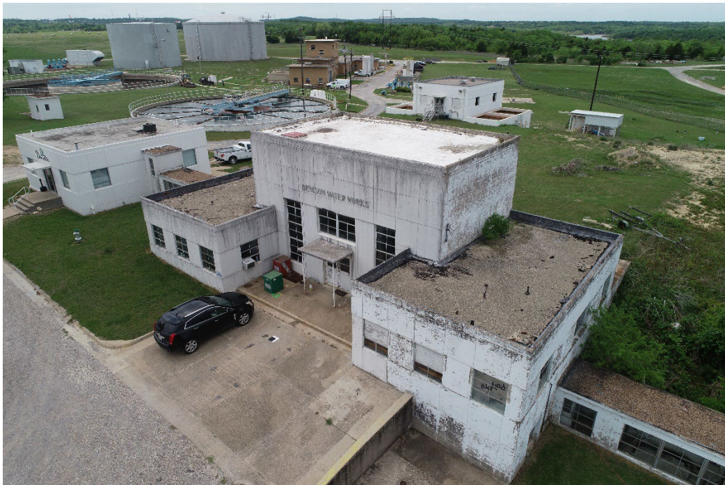
Photograph 2: Filter Building No. 0 with adjoining Pump Station and Chemical Building - Originally constructed in 1941, decommissioned in 1993.
