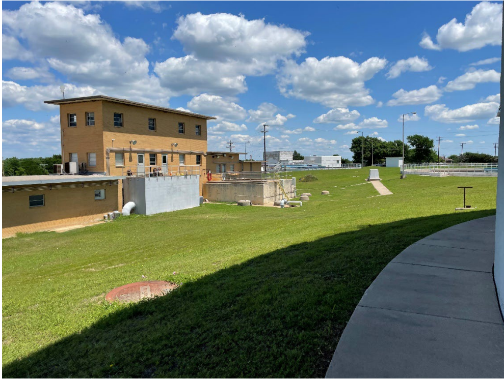
Photograph 3: Filter building No.2 – Originally constructed in 1978.
