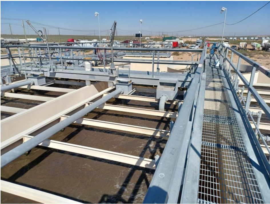
Flow Equalizer Basins in the center of the facility, photo taken facing NW
