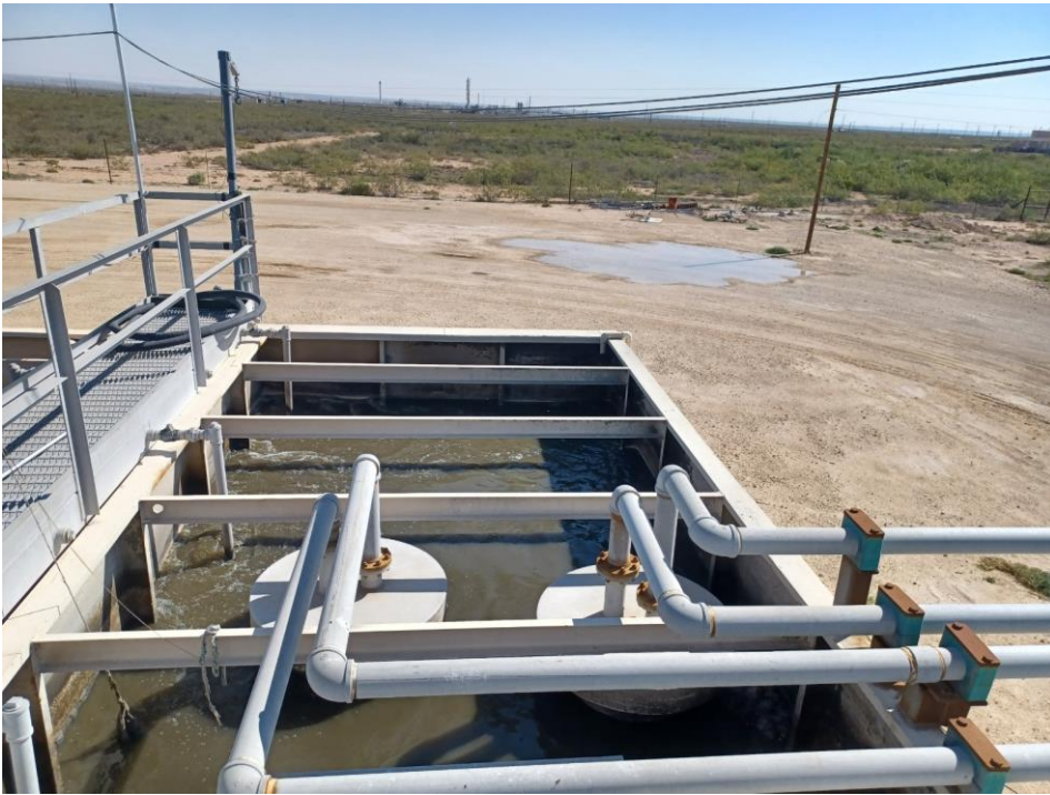
Flow Equalizer Basin No. 1 facing NE on the SE of the facility
