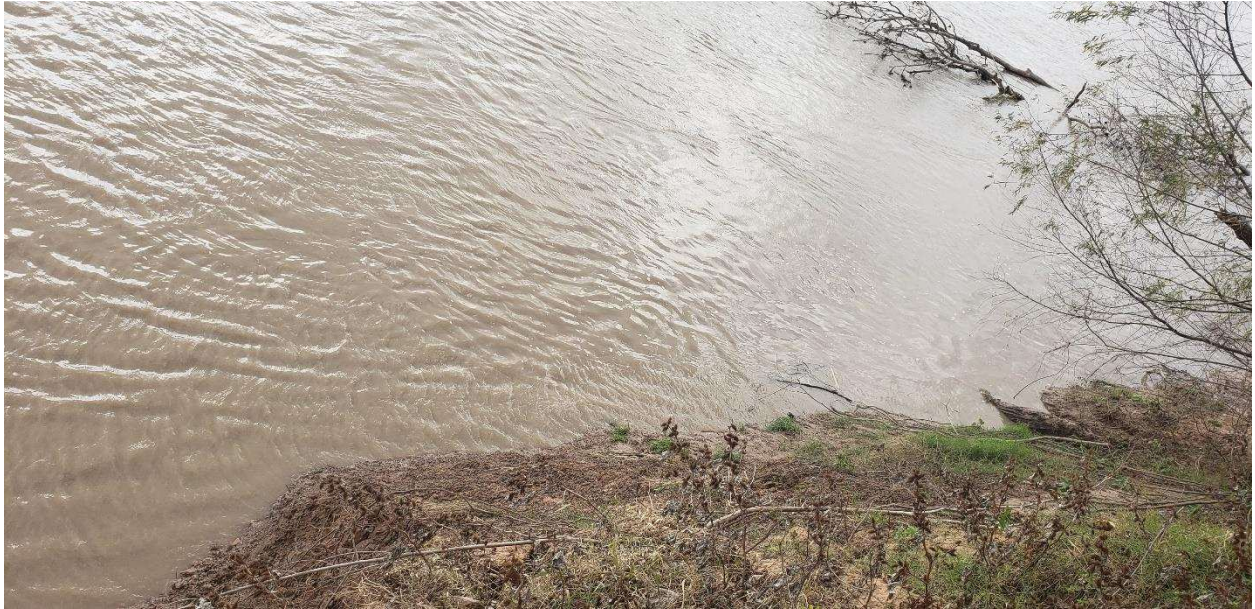
Photo 3 – Proposed Richmond East WWTP Outfall Location To Brazos River Segment 1202 (looking south)
