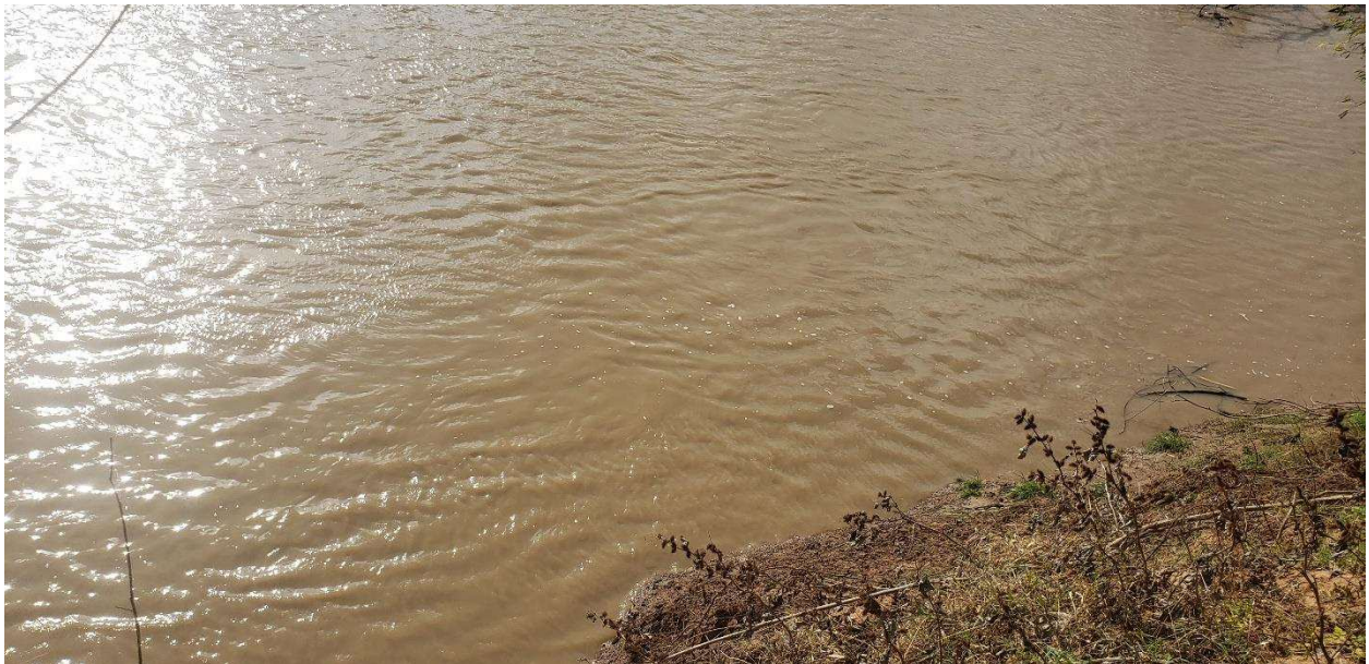
Photo 4 – Close-Up Proposed Richmond East WWTP Outfall Location To Brazos River (looking south)
