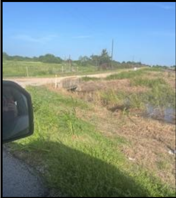
PICTURE 9 DOWNSTREAM DITCH CULVERT AT OLD PORT LAVACA RD (FACING NE)
