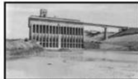
"Construction of Lake Texoma Intake Structures"
