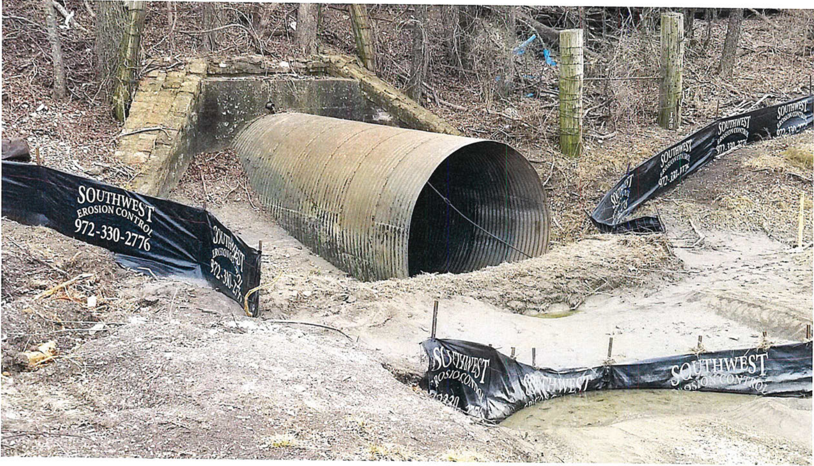
Photograph A – Upstream side of existing culvert
