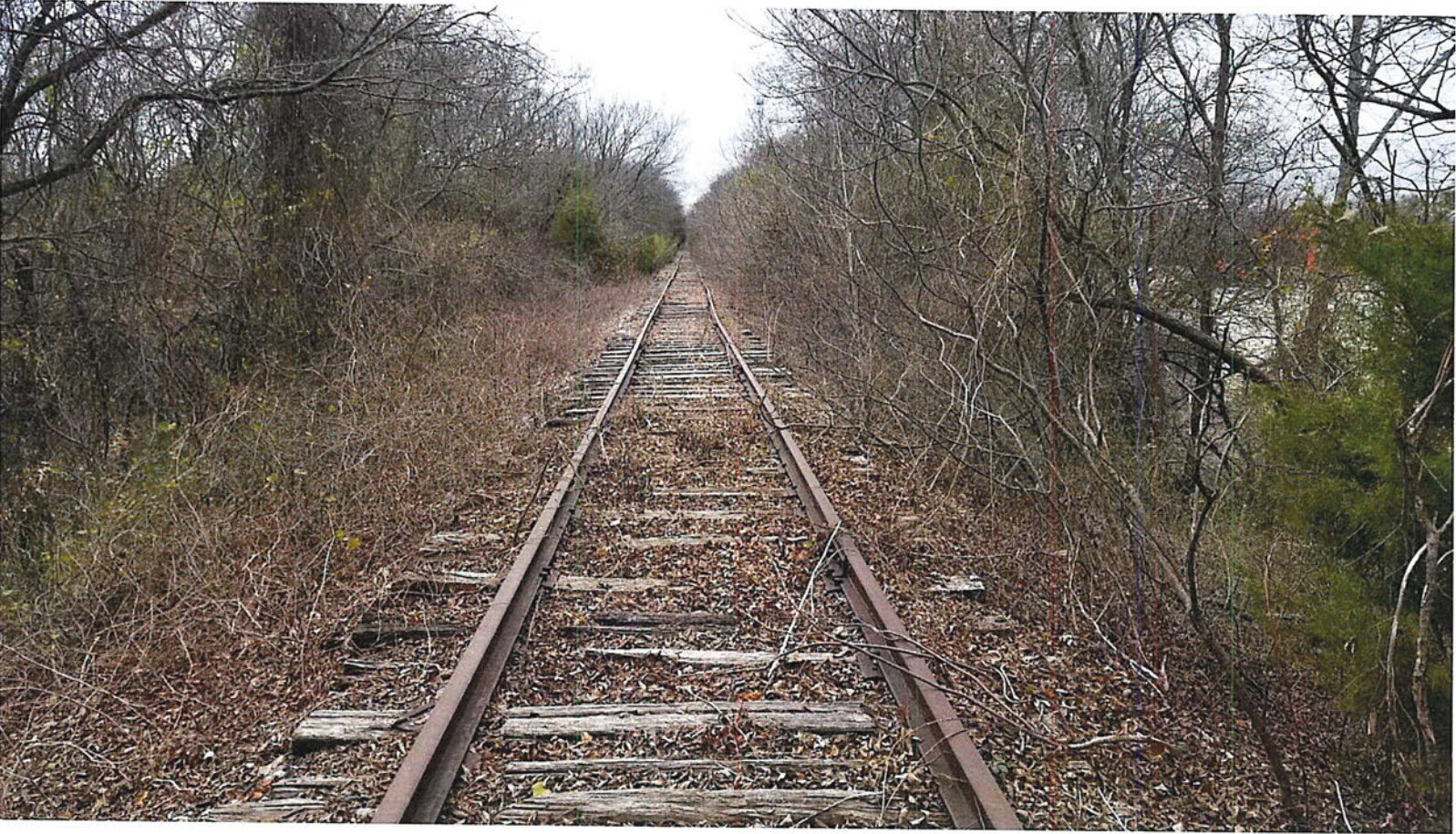
Photograph D – Existing rail road facing southwest
