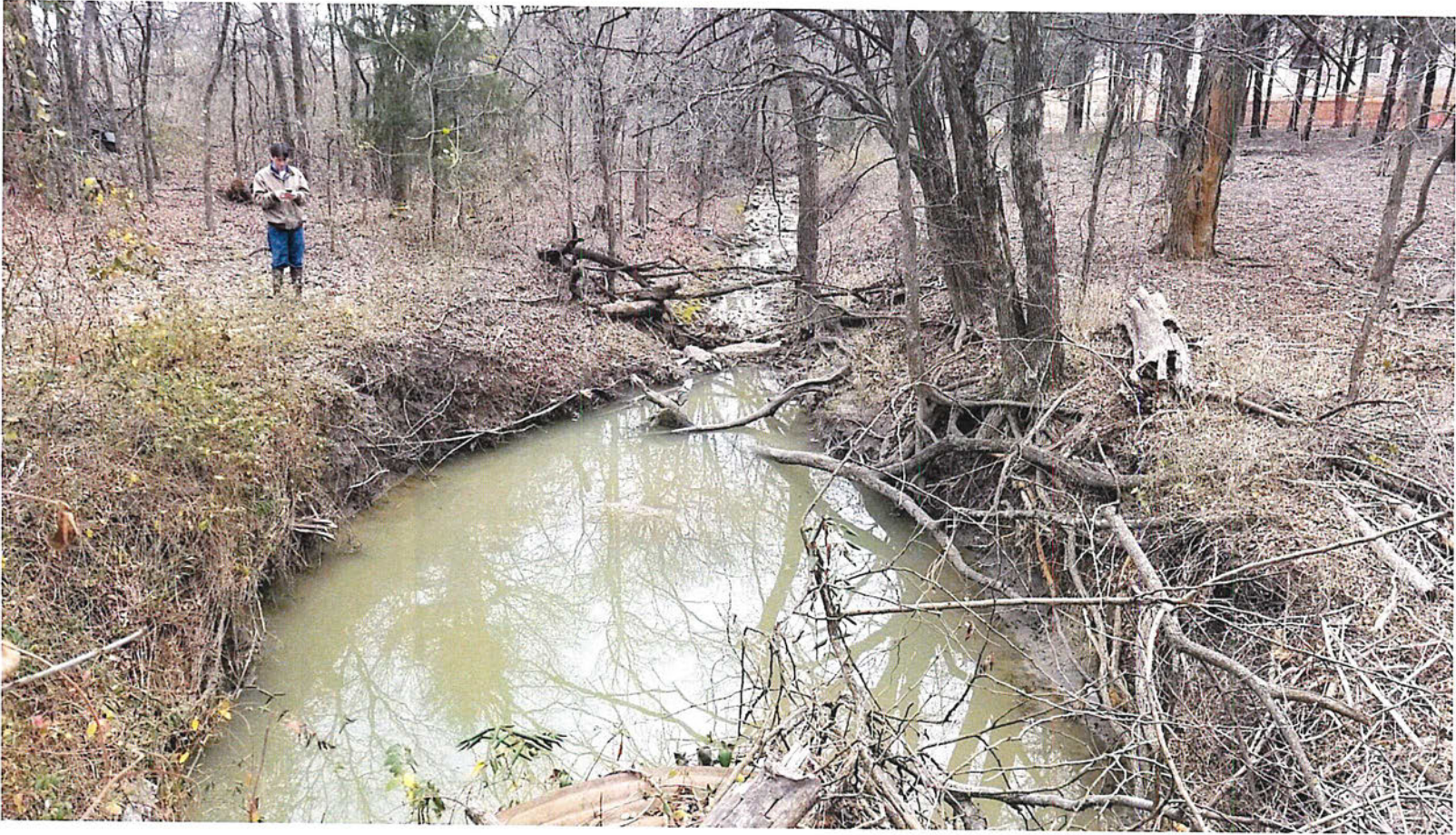
Photograph H – Downstream ripple pond from culvert headwall
