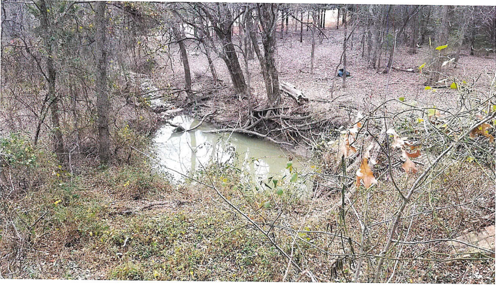
Photograph G – Facing downstream culvert from railroad
