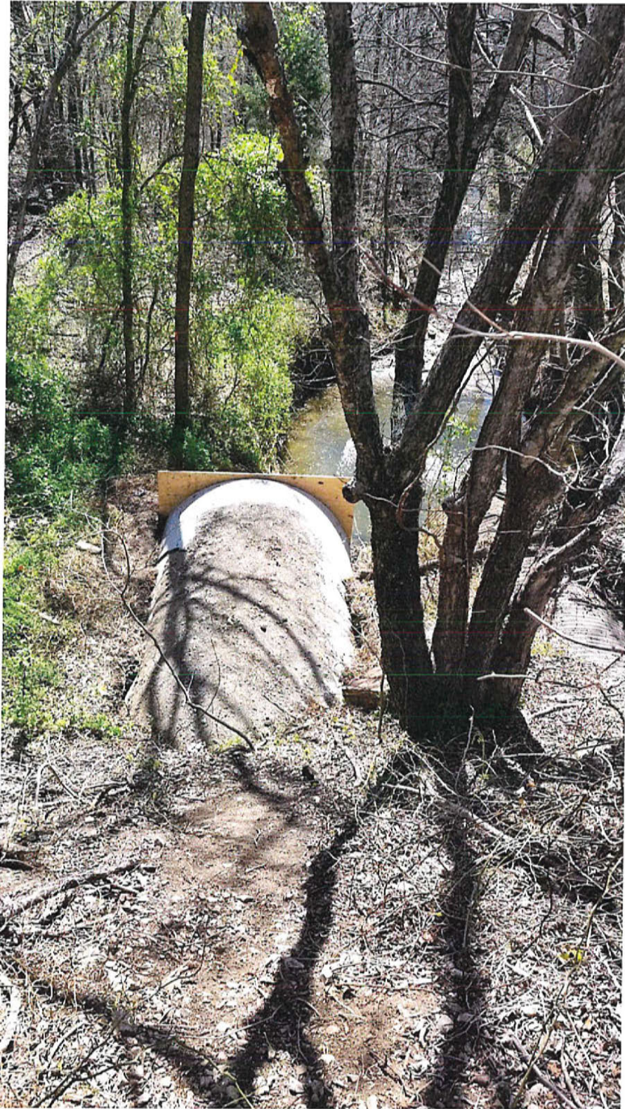
Photograph K – Facing downstream from railroad with new RCP
