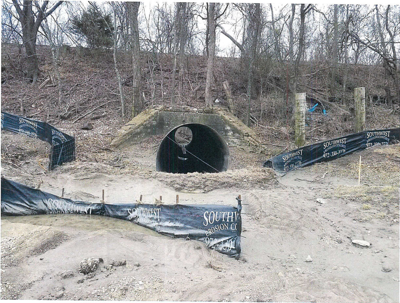
Photograph C – Upstream side of existing culvert
