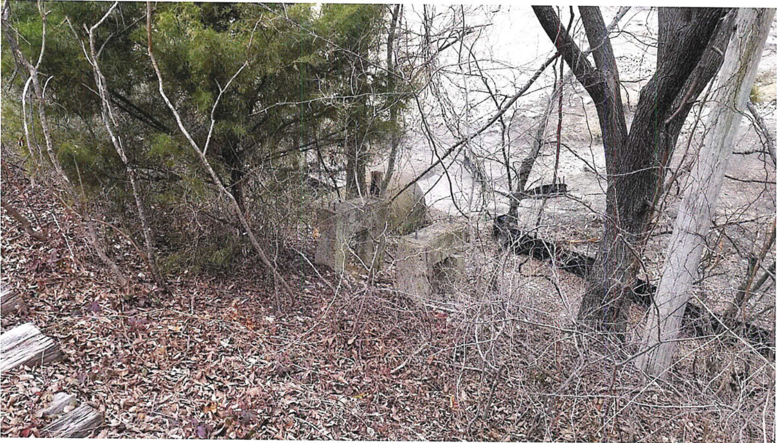
Photograph E – Facing upstream culvert from railroad
