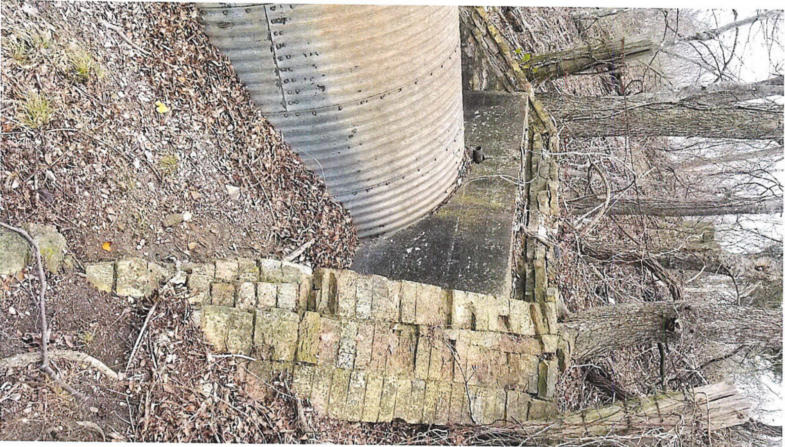
Photograph B – Upstream side of existing culvert headwall
