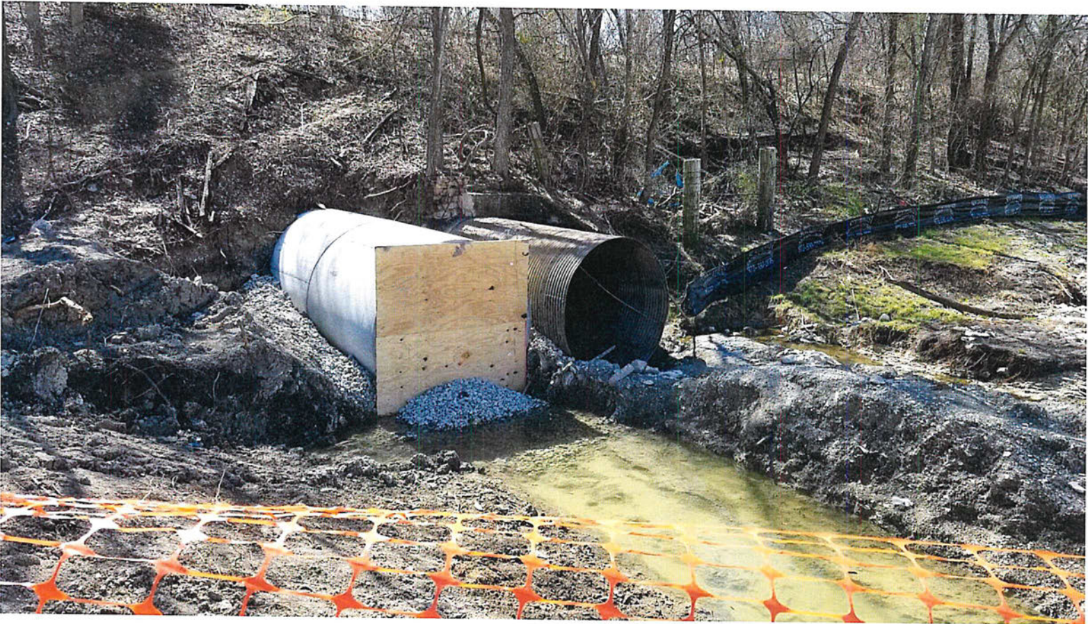
Photograph J – Upstream side of culvert with new RCP
