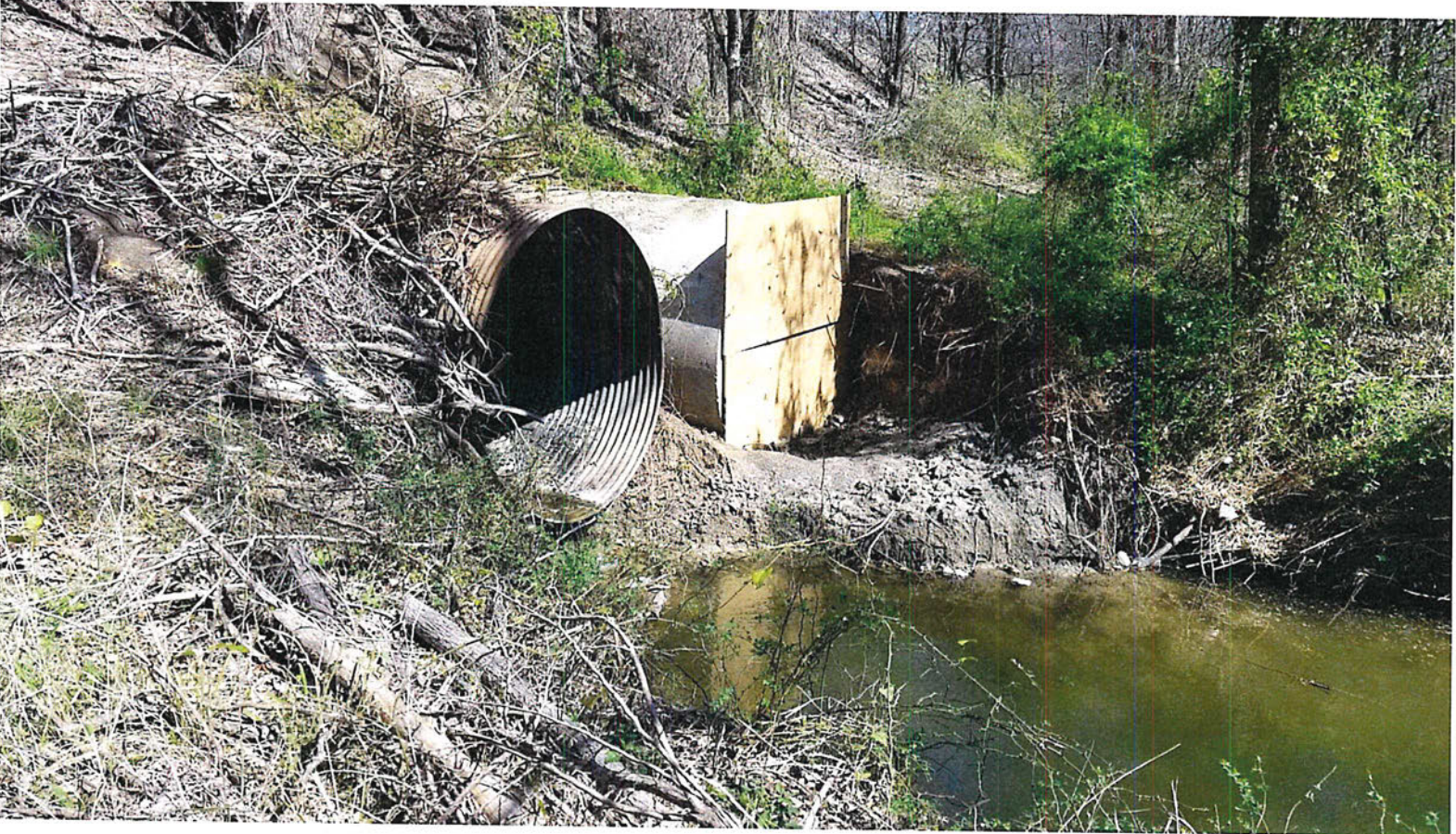
Photograph L – Downstream side of culvert with new RCP
