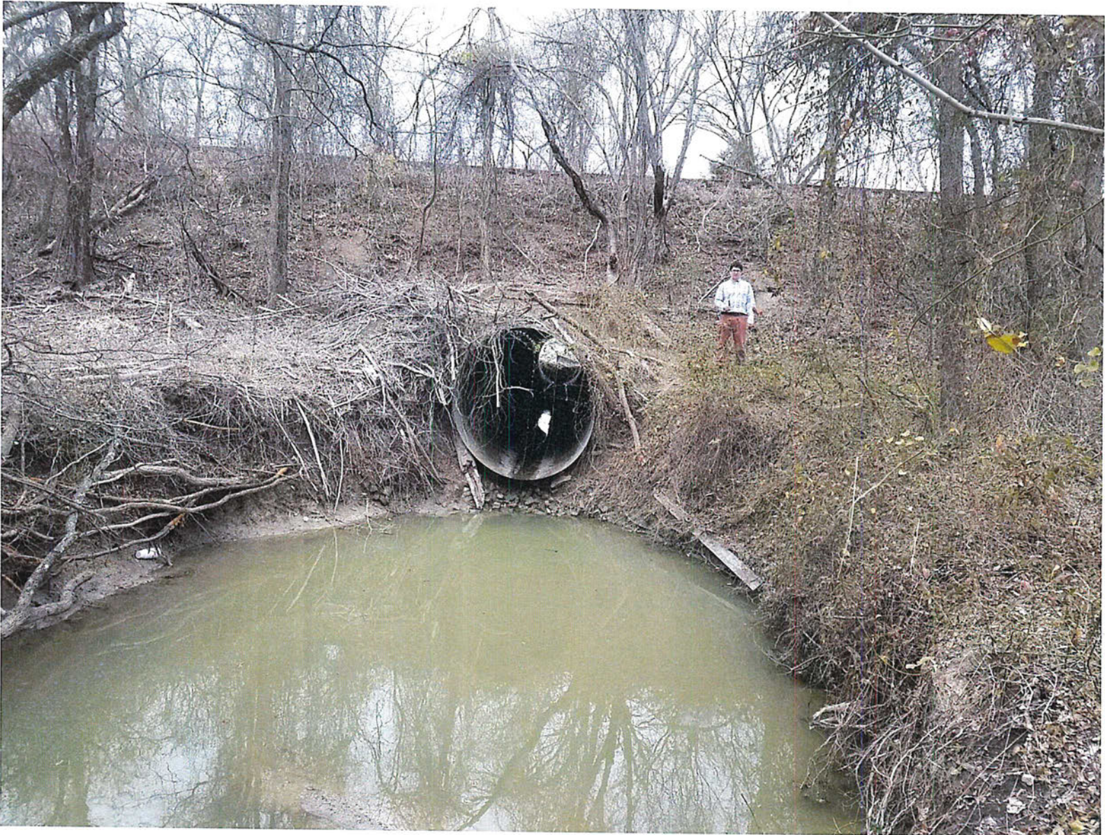
Photograph 1 – Downstream side of culvert
