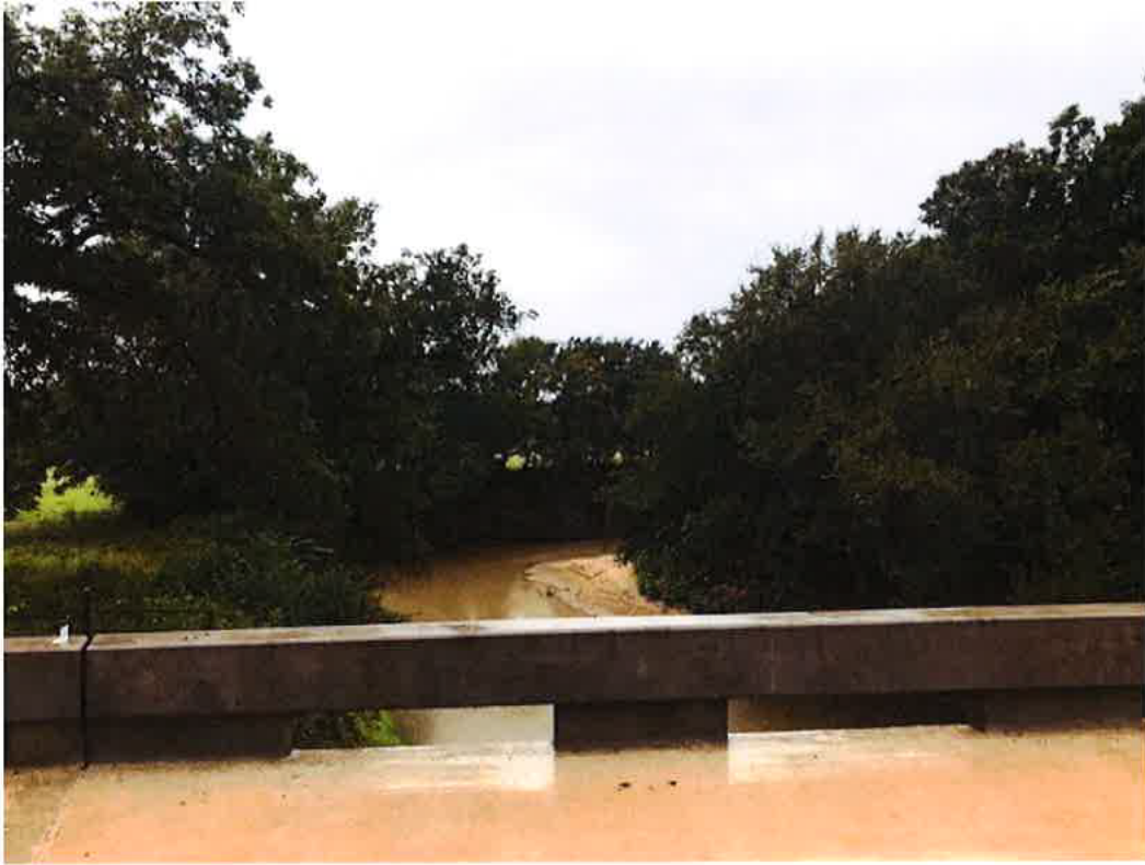
1.) Upper Limit of Diversion Reach #1 Facing Upstream
