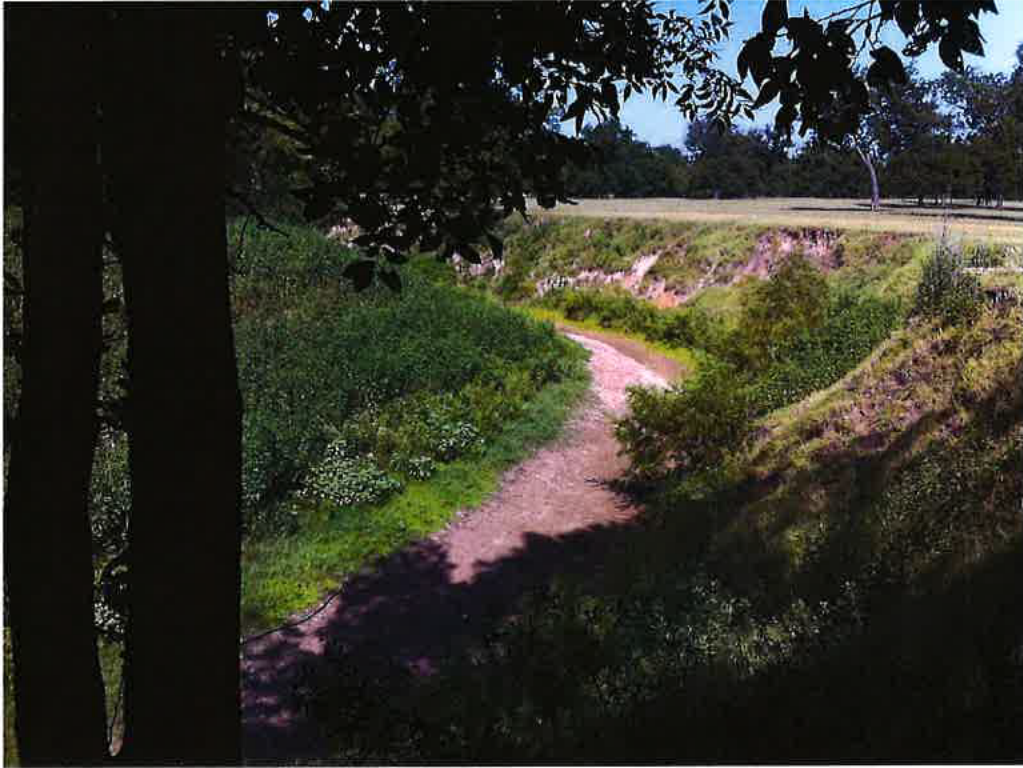
3.) Lower Limit of Diversion Reach #1 Facing Upstream
