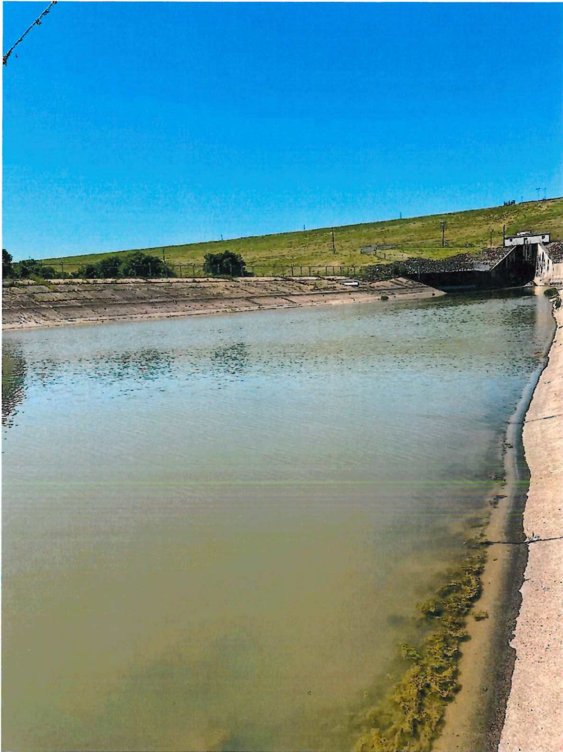
Photo 3 – Lake Brazos upstream of Airport Road, looking upstream of the proposed diversion point towards Lake Waco dam.
