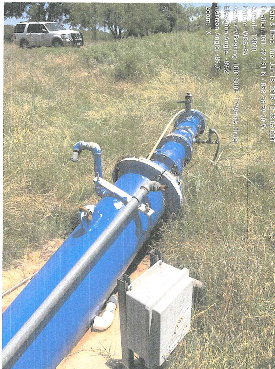
Figure 4 – City of Goldthwaite's installed and operating diversion infrastructure (pump, meter, and pipeline)
