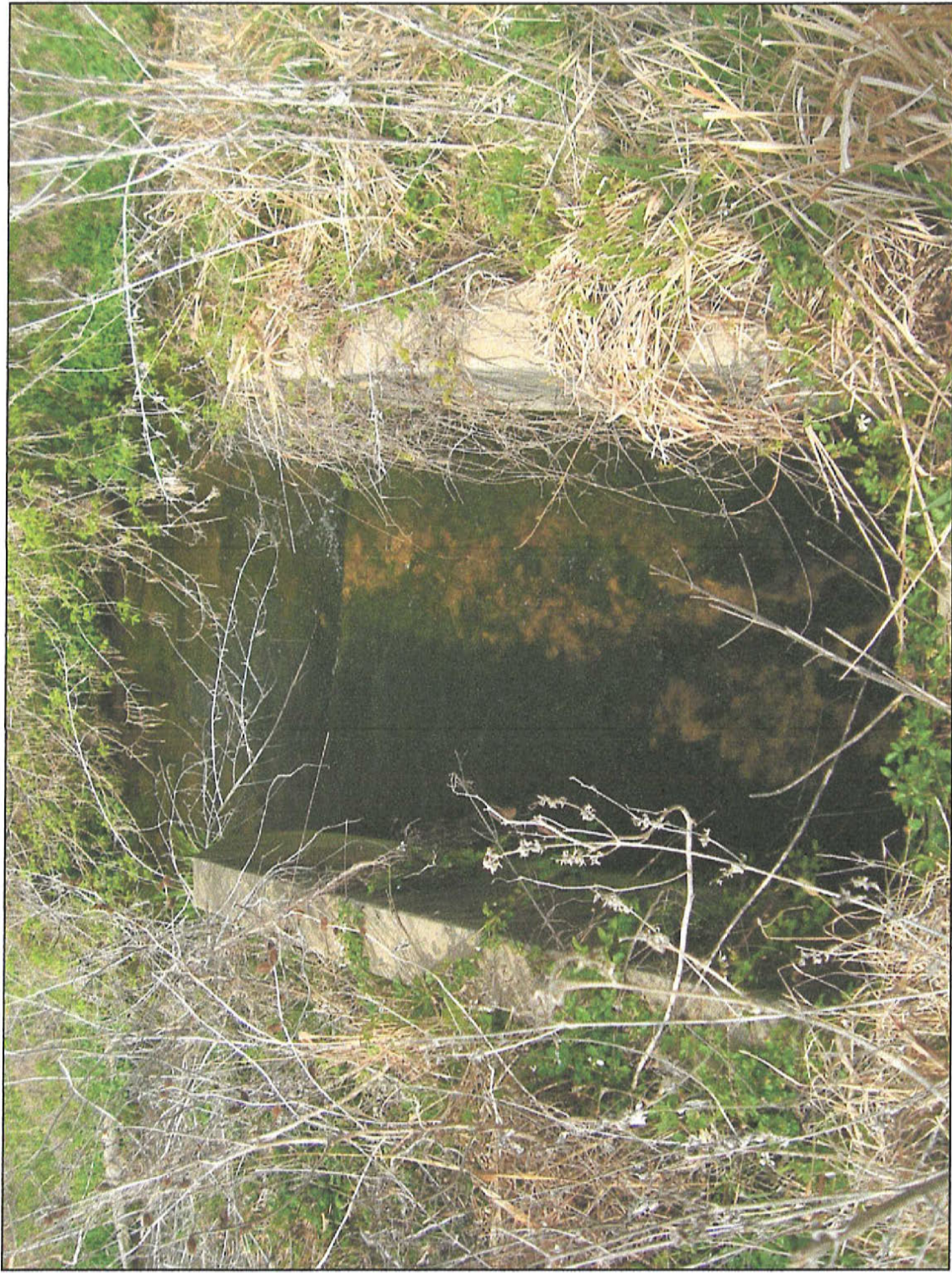
Robinson Creek WWTP - Outfall
