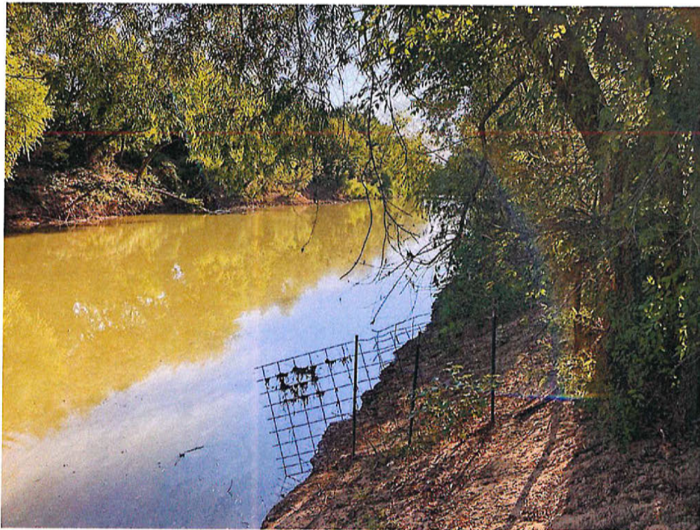
Photo 10: (Reach C-C') Downstream Limit C' Looking Downstream
