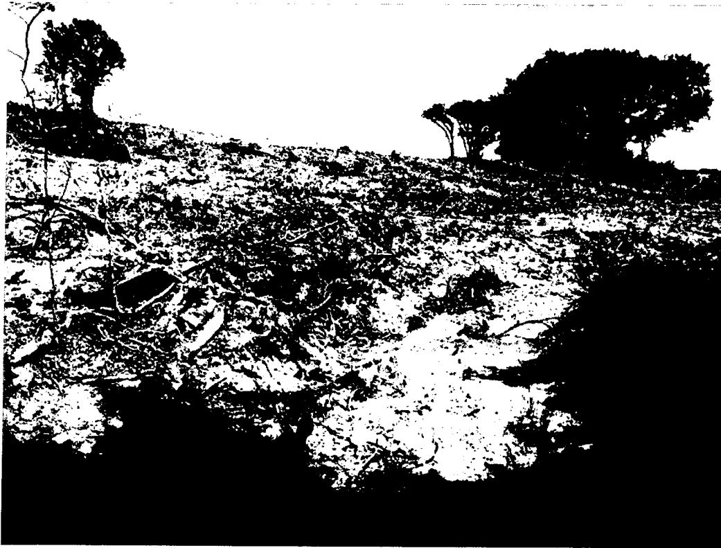
Photo 23: (Reach E-E') Downstream Limit E' Looking Upstream
