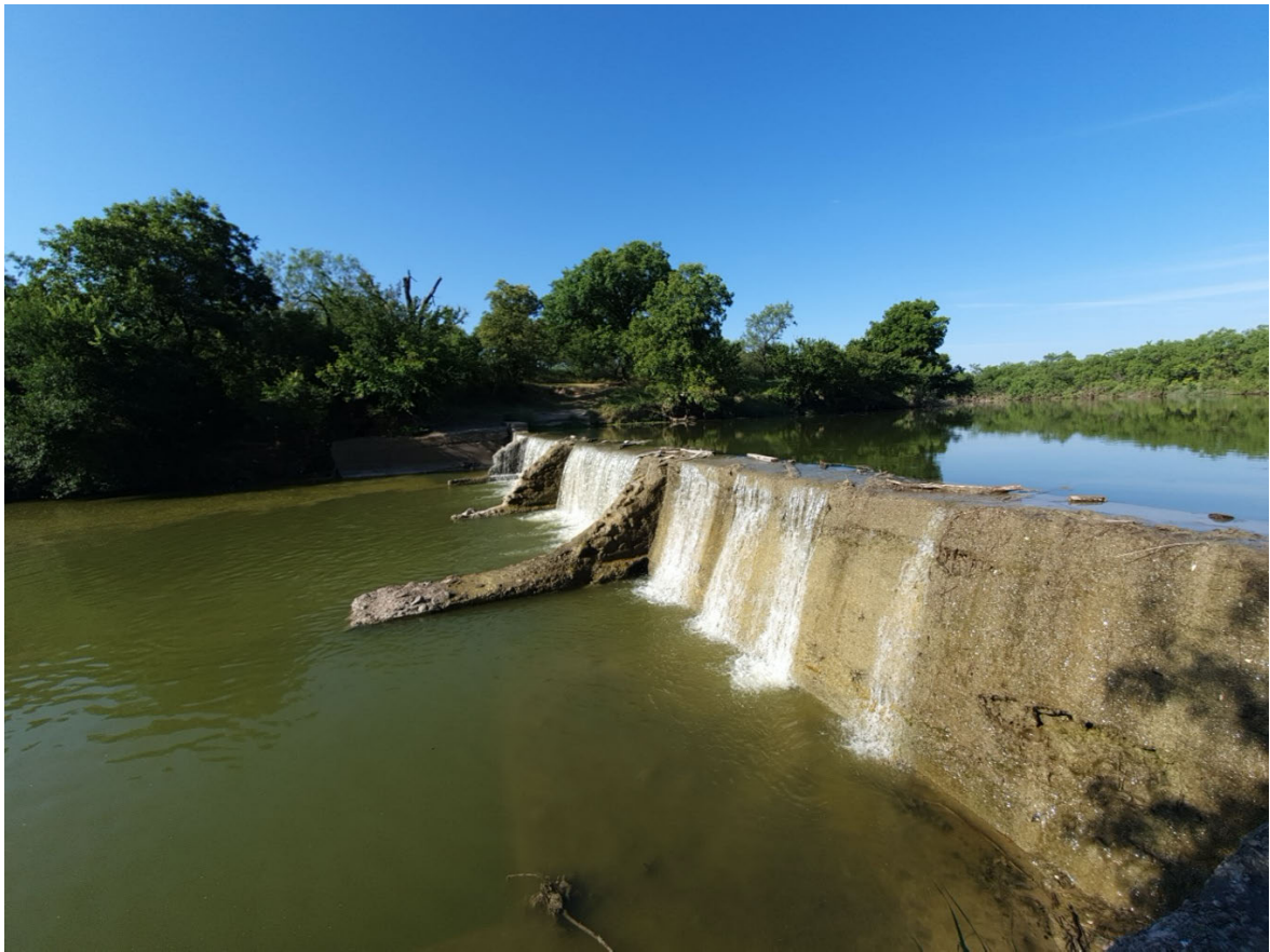
Photo 1 - Discharge Point Immediately Downstream of Dam (COA 14-1337)
