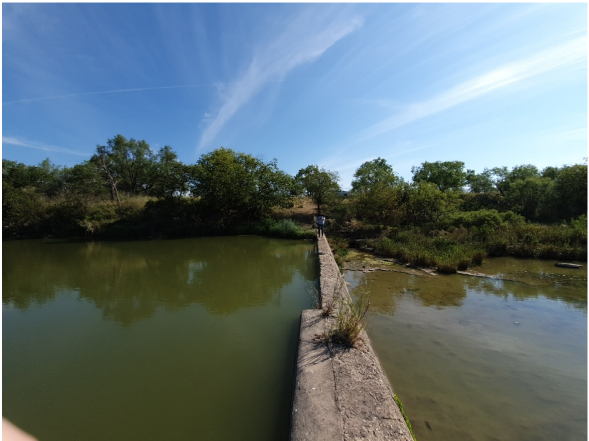
Photo 10 – Diversion Point in Reservoir Upstream of North Section of Dam
