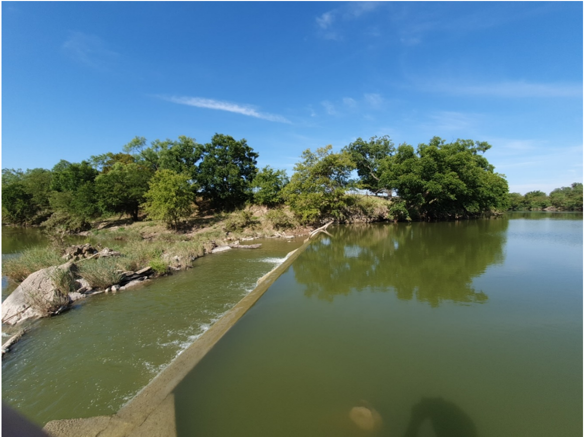
Photo 9 –South Overflow Section of Dam near Diversion Point
