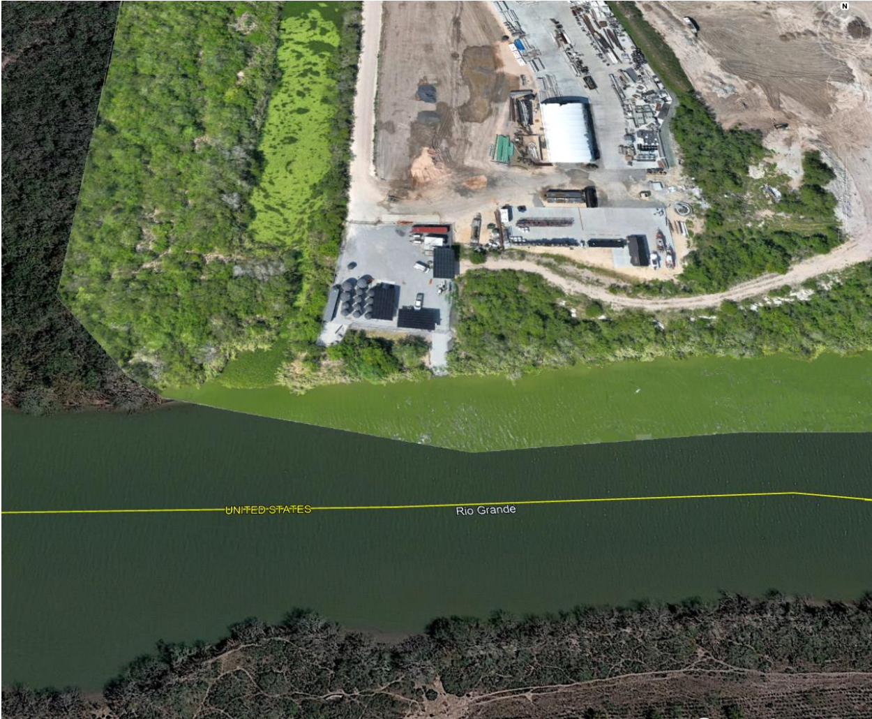
Diversion point aerial
