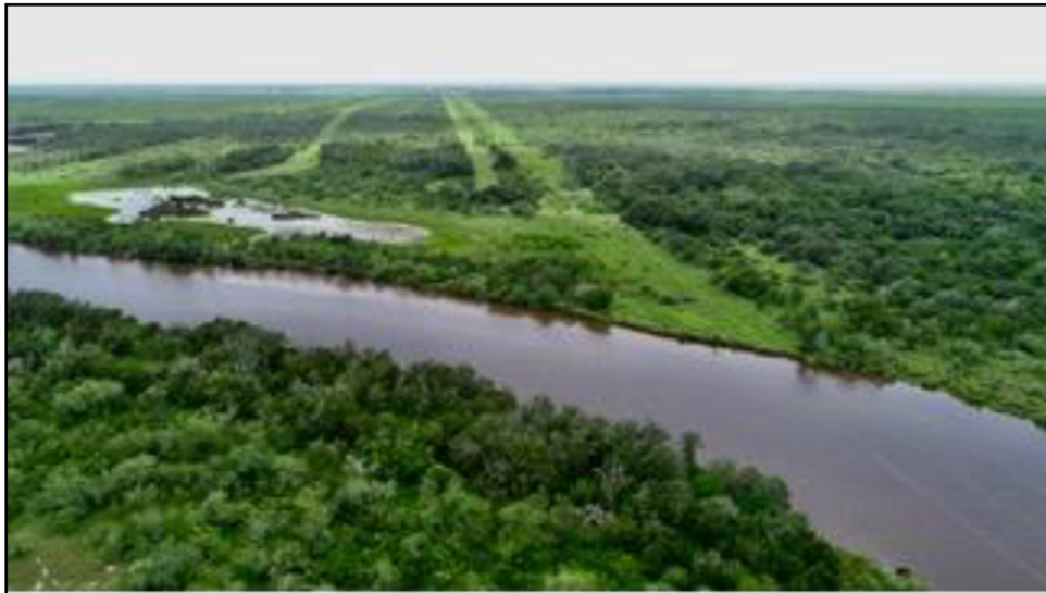
Figure 4. View west at the water diversion reach.
