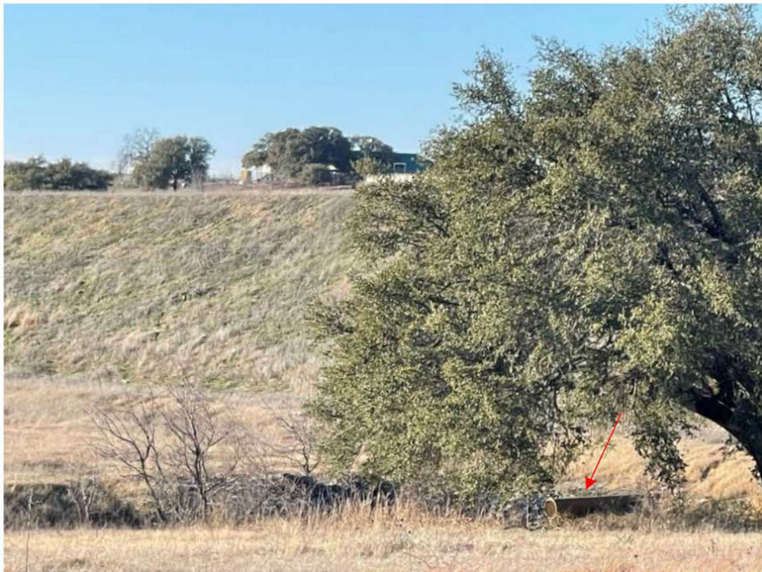
Photo 7: Back side of Site 25 Dam facing principal spillway water outlet
