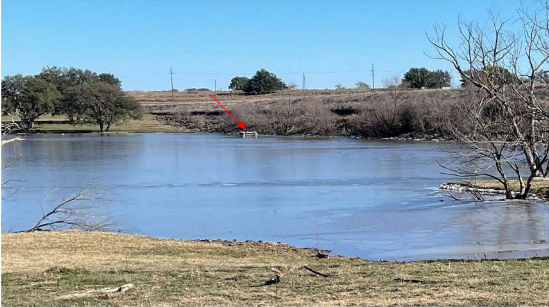
Photo 6: Reservoir side of Site 25 Dam facing principal spillway water inlet
