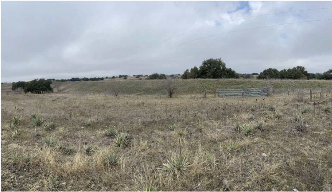
Photo 1 (Panoramic): East end looking northwest down the length of Site 25 Dam
