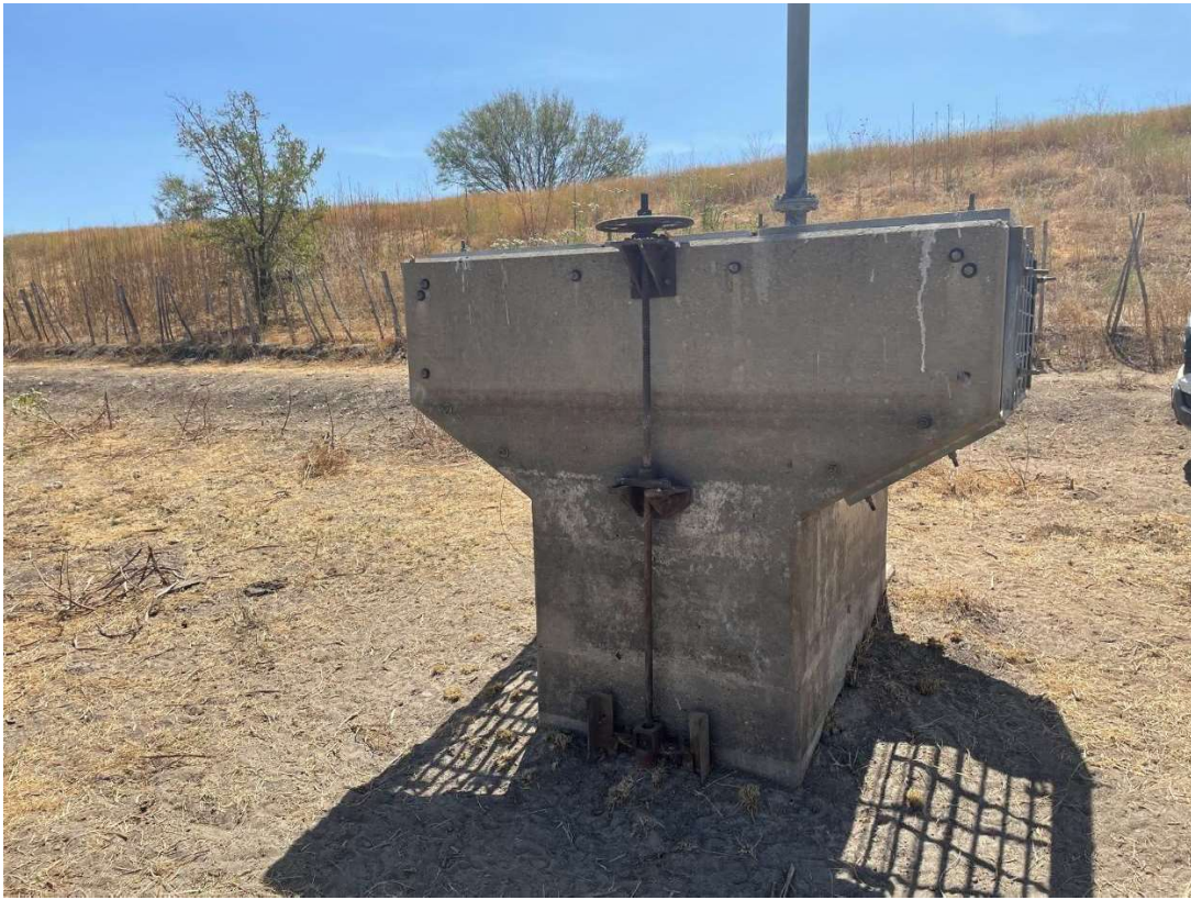
Photo 14: Reservoir side of Site 26 Dam facing principal spillway water inlet
