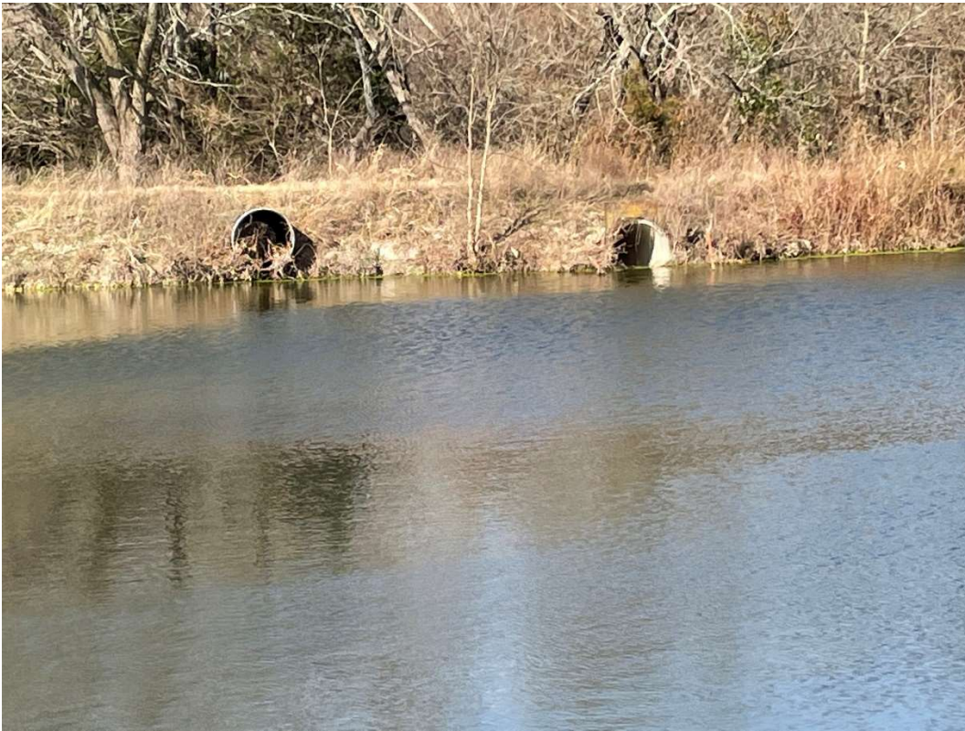
11-DAM WITH 2-18" SPILLWAY PIPES
