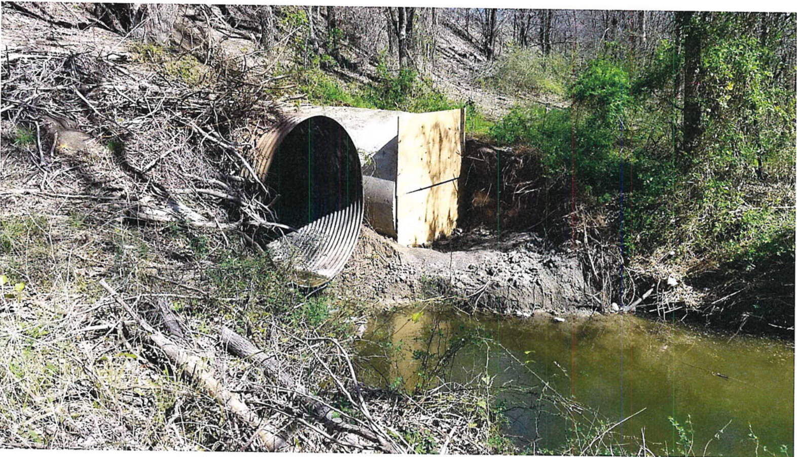
Photograph L – Downstream side of culvert with new RCP
