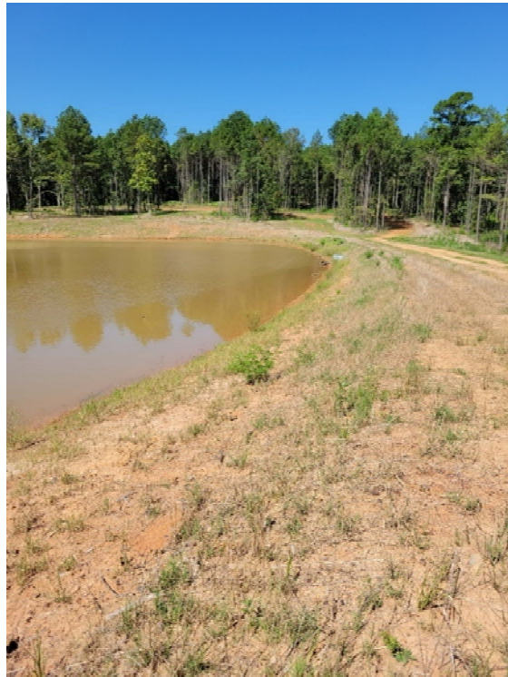
Photo 2. Viewing the constructed road and dam on the north side of the impoundment on the northern part of the property from the east facing west.
