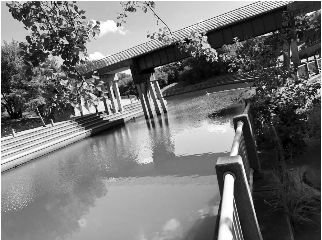
Map Number 57: Downstream Limit for Diversion Reach White Oak Bayou #3 looking downstream.
