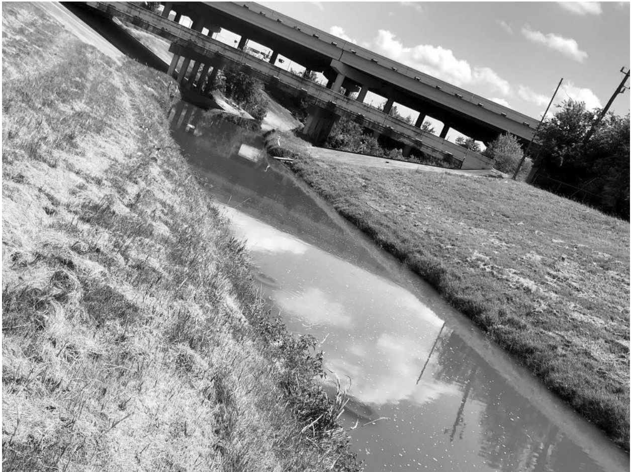
Map Number 36: Upstream Limit for Diversion Reach Sims Bayou #1 looking downstream.
