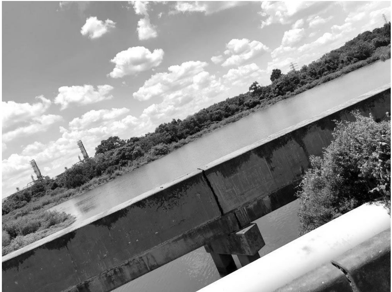
Map Number 34: Downstream Limit for Diversion Reach Hunting Bayou #1 looking downstream.
