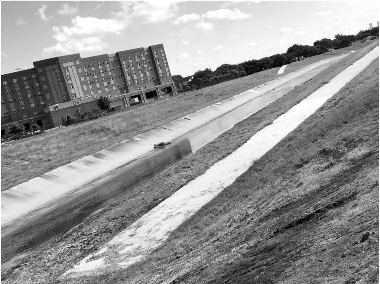
Map Number 6: Downstream Limit for Diversion Reach Brays Bayou #2 and Upstream Limit for Diversion Reach Brays Bayou #3 looking downstream.
