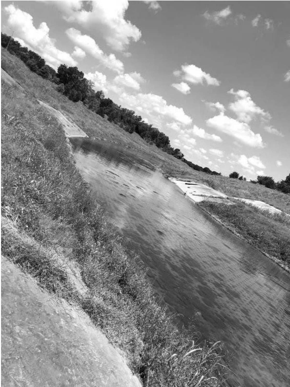
Map Number 39: Downstream Limit for Diversion Reach Sims Bayou #2 and Upstream Limit for Diversion Reach Sims Bayou #3 looking upstream.
