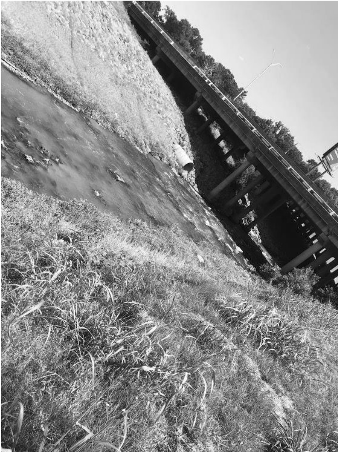
Map Number 18: Downstream Limit for Diversion Reach Greens Bayou #4 and Upstream Limit for Diversion Reach Greens Bayou #5 looking downstream.
