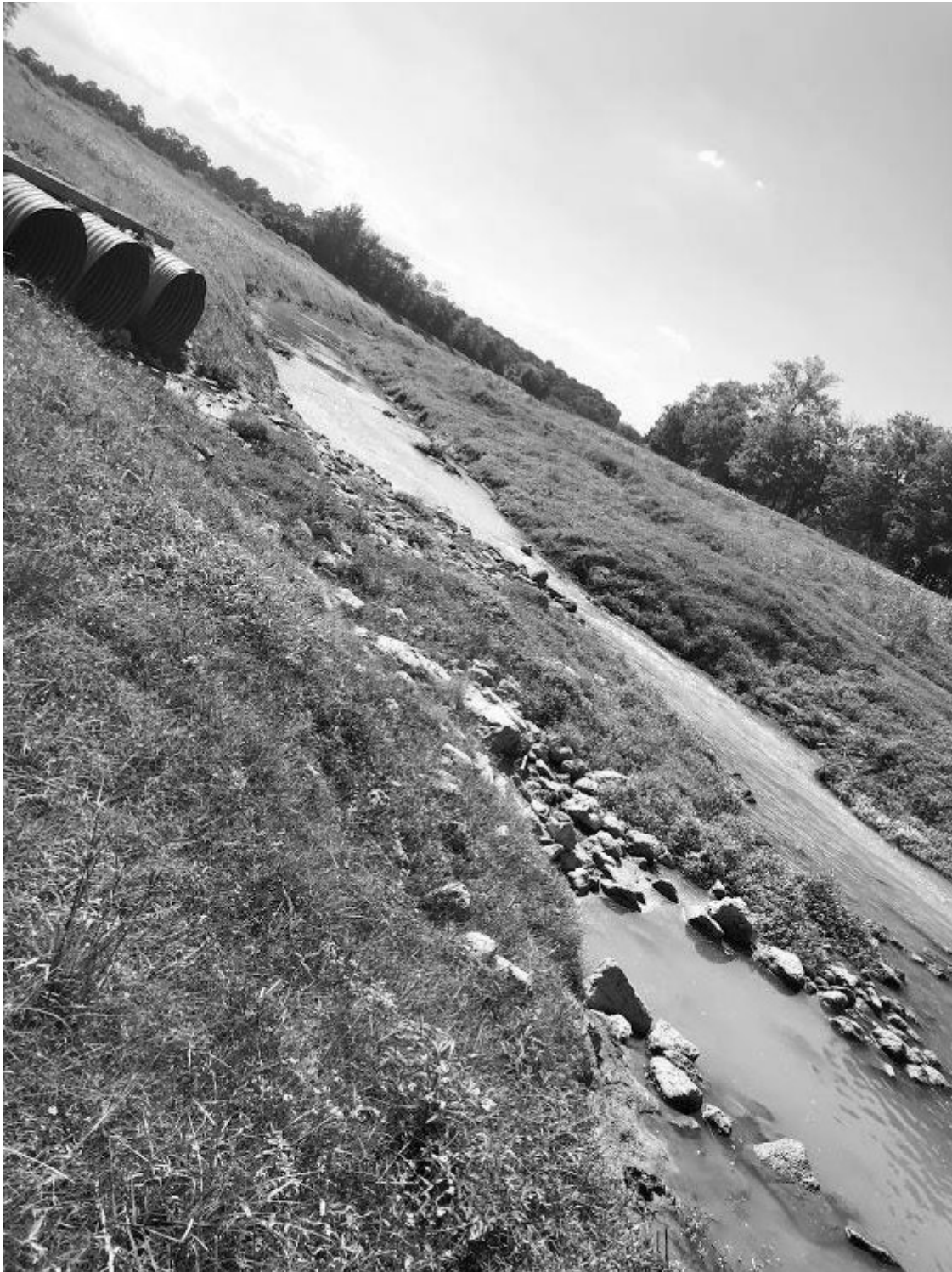
Map Number 19: Downstream Limit for Diversion Reach Greens Bayou #5 and Upstream Limit for Diversion Reach Greens Bayou #6 looking upstream.
