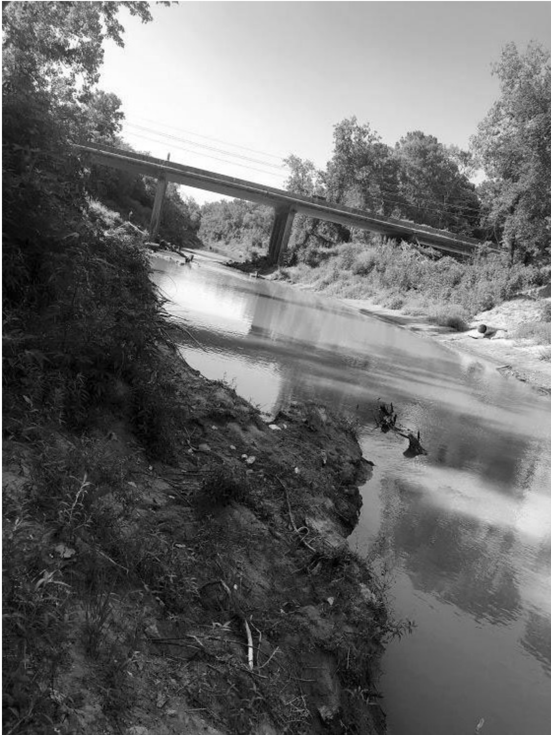
Map Number 23: Downstream Limit for Diversion Reach Greens Bayou #7 and Upstream Limit for Diversion Reach Greens Bayou #8 looking upstream.
