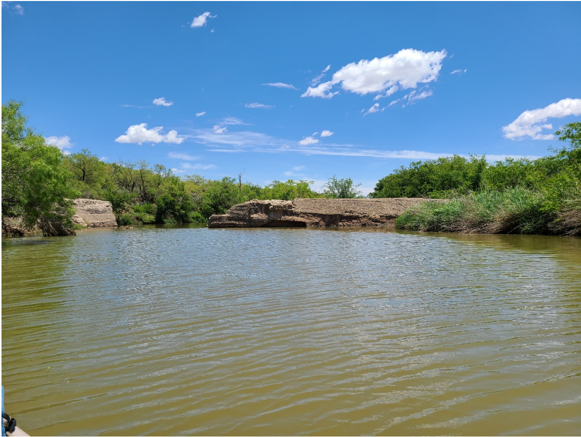
Photo 5 – Failed Dam Structure within Conveyance Reach
