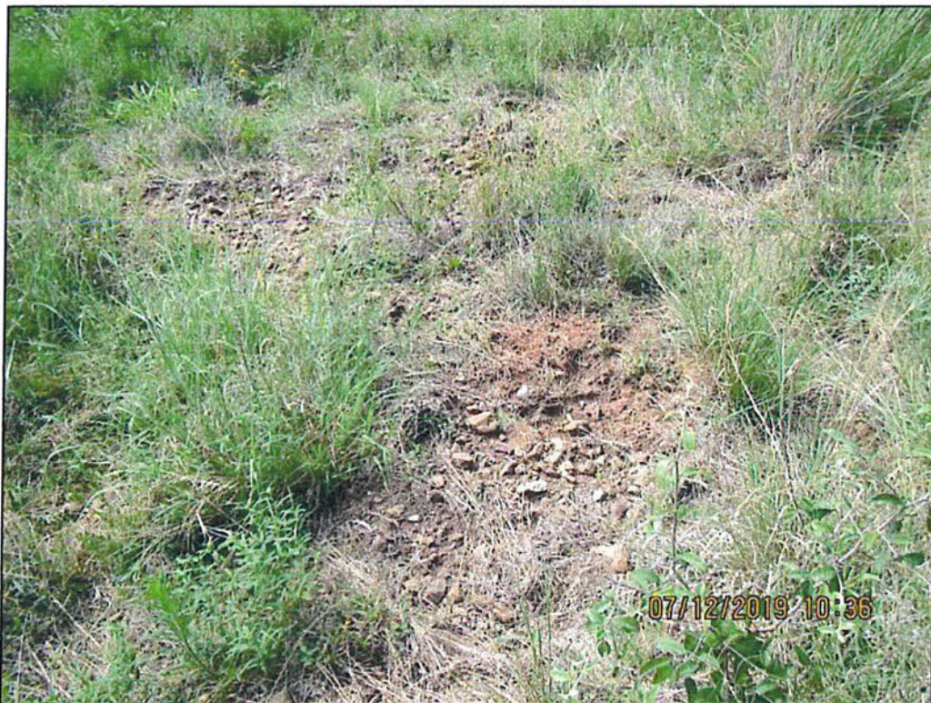
Photo 14 – Downstream slope. Near right end. Looking upstream and to right. Note hog damage.
