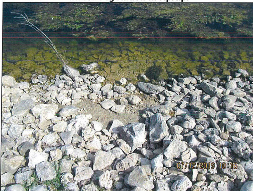
Photo 6 – Upstream slope. Displaced riprap and exposed embankment.
