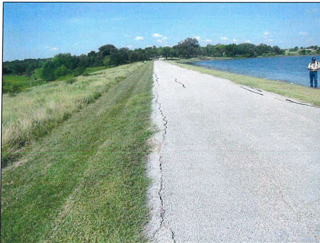
Photo 3 – Crest. Looking right. Note asphalt concrete cracking.
