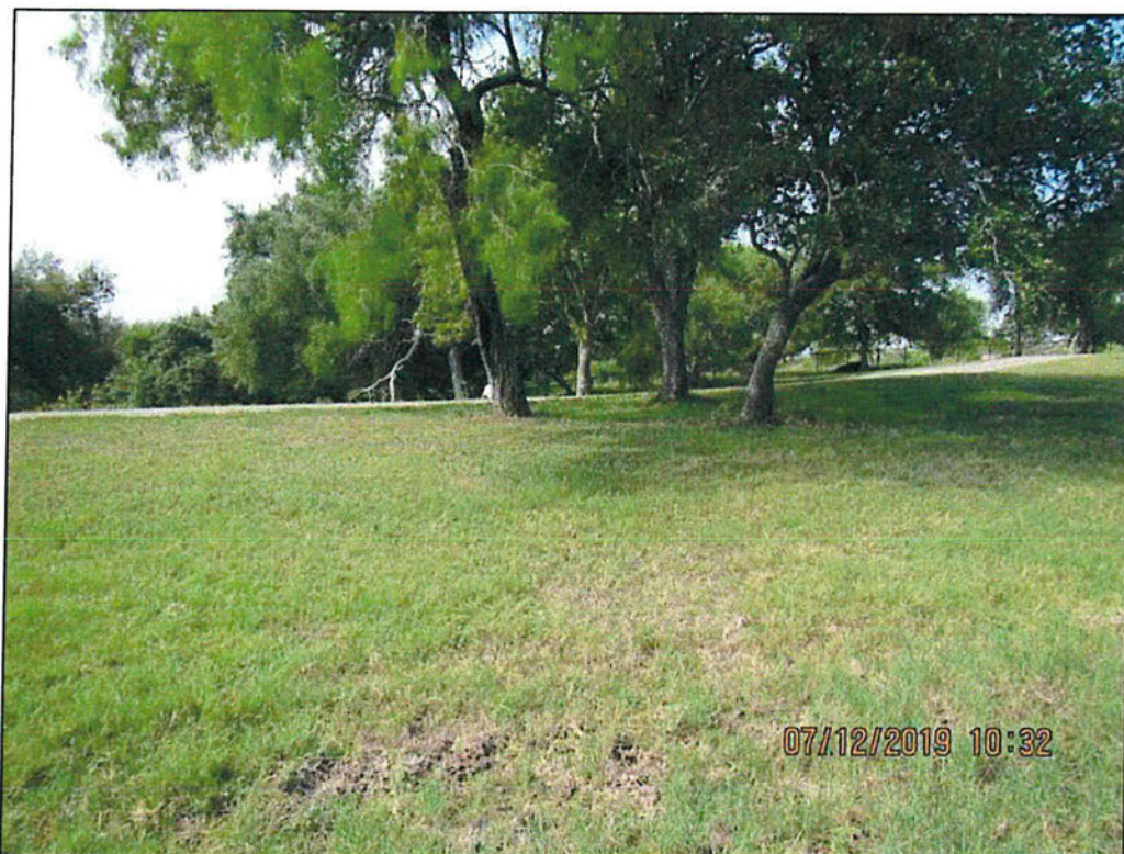
Photo 29 – Emergency spillway approach. Looking downstream. Note large trees in spillway flowpath.
