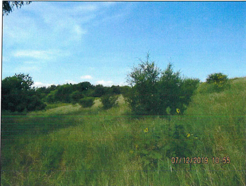
Photo 13 – Downstream slope. Mid embankment. Looking right. Note trees and brush.
