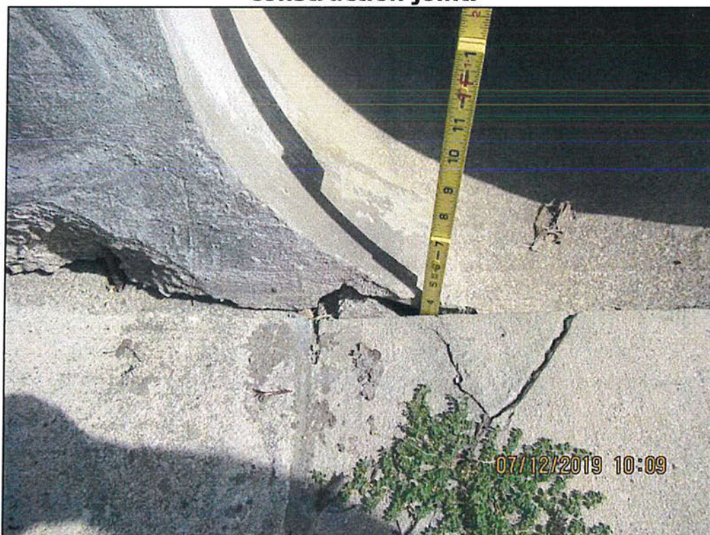
Photo 22 – Service spillway. Culvert pipe outlet at right end. Note spalling, cracks, voids, open joints, exposed reinforcing steel.
