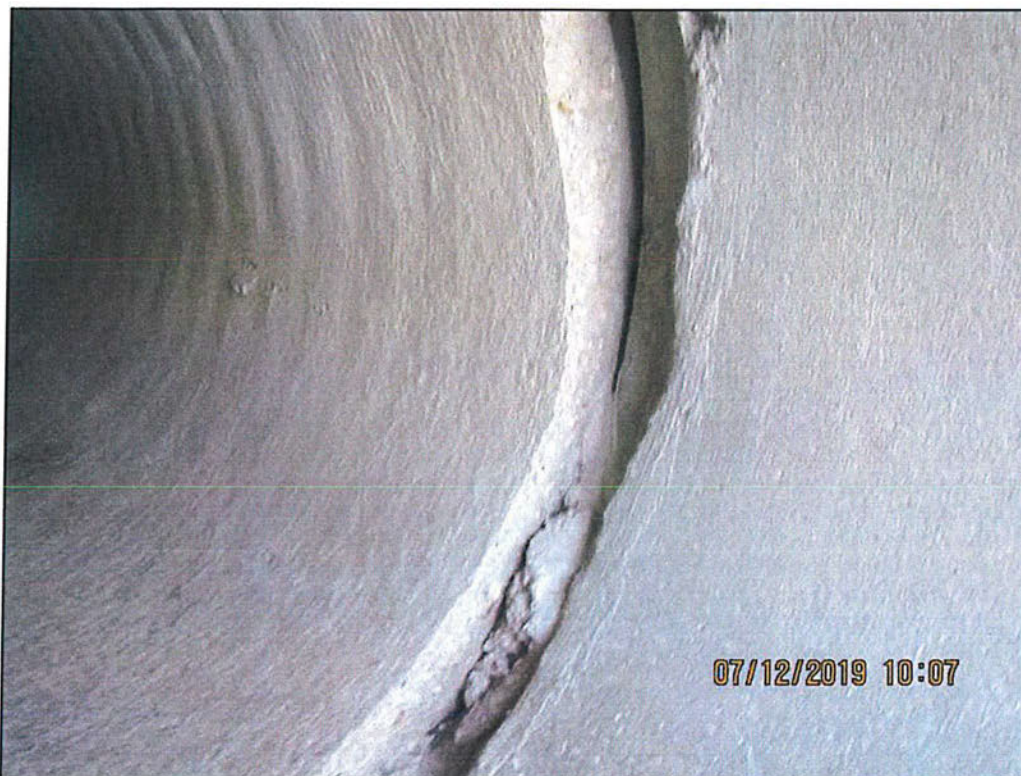
Photo 21 – Service spillway. Upstream side. Note typical gaps in construction joint.
