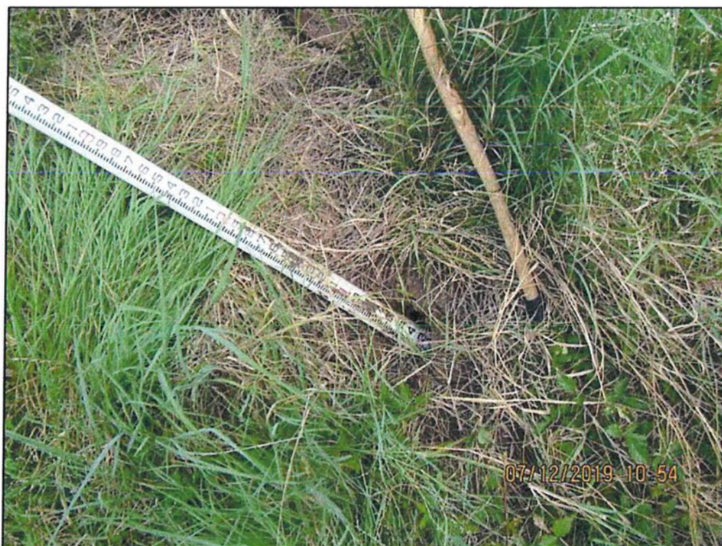
Photo 18 – Downstream slope. Typical animal burrow.
