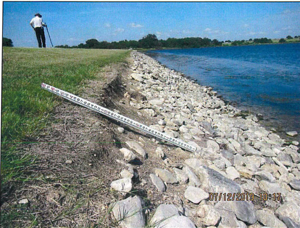
Photo 7 – Upstream slope. Looking right. Note displaced riprap and benching erosion.
