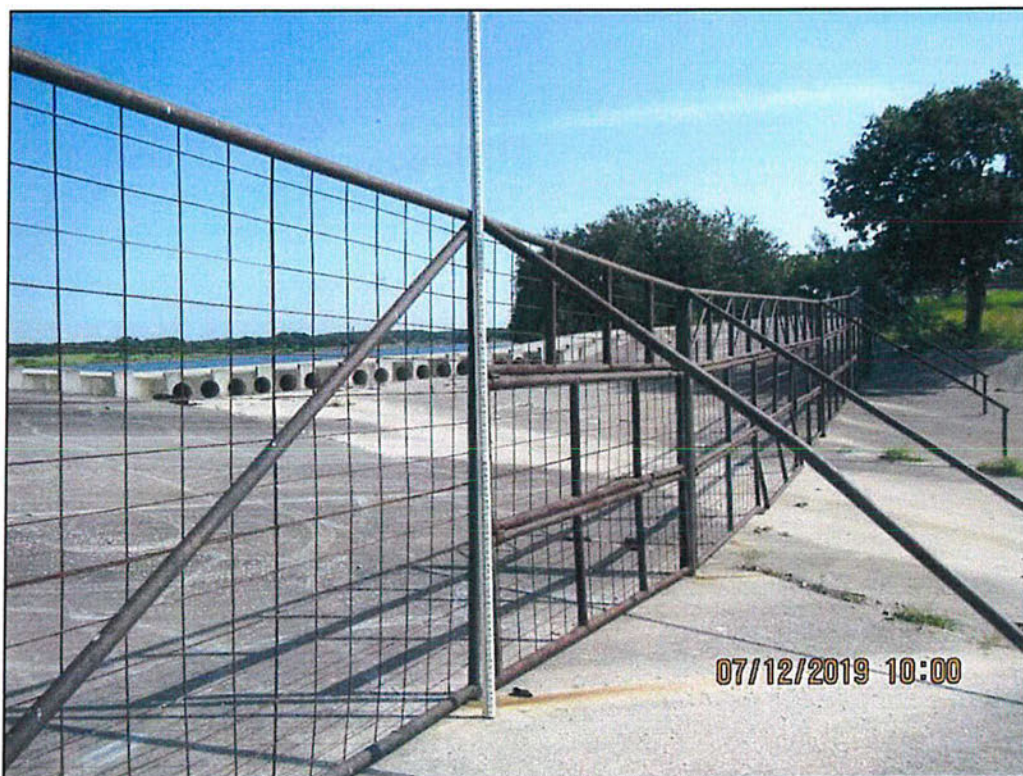
Photo 23 – Service spillway. At right side looking upstream. 8-foot fence with flap gate sections. Note corrosion.
