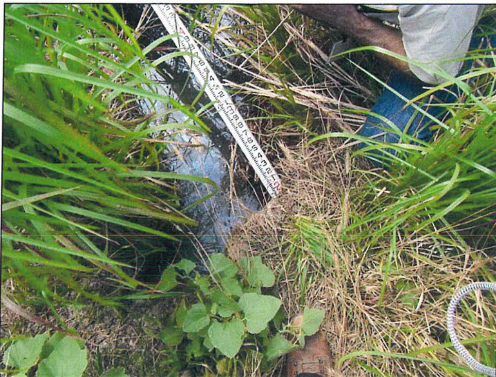
Photo 17 – Downstream toe. Seepage. Note animal activity.
