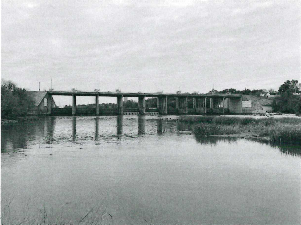
Photograph 2: Looking upstream, just downstream of the Upstream Diversion Limit, Longhorn dam. Showing area downstream of the Upstream Diversion Limit.
