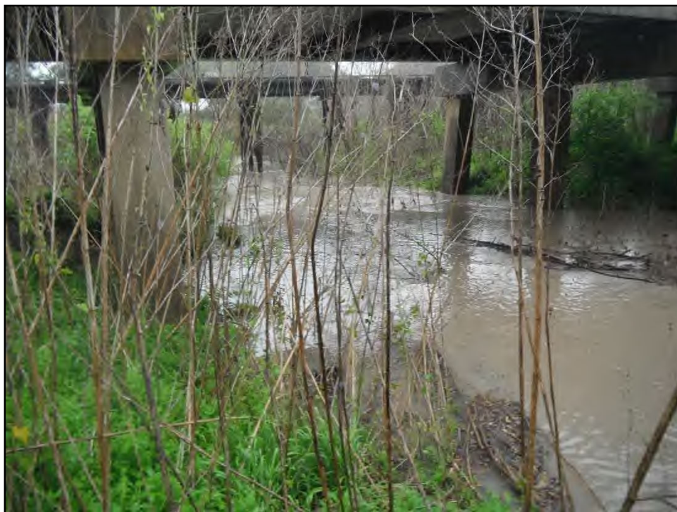
Photo 2. Photograph on the north side of SAR Transect 2 taken during the stream assessment, facing south towards the existing concrete flume and timber bridge.
