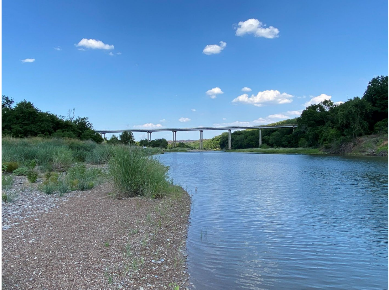
Photograph at Diversion Reach 2 (East Property Line) Looking East (Downstream). View of FM 4 Bridge Over the Brazos River.
