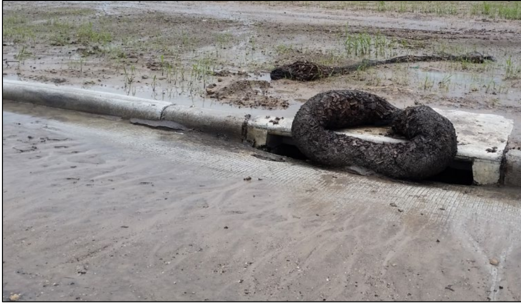
Figure 53. Example of a failing stormwater BMP; photo taken just north of the Highland Bayou watershed.
