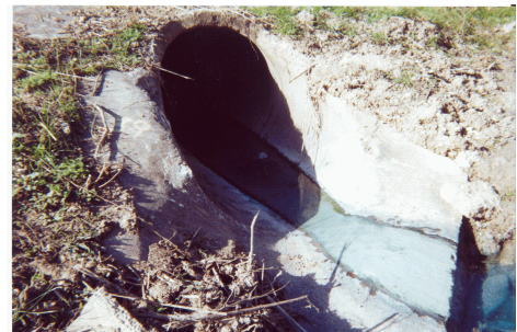
Figure 5. Source of blue water was a car wash facility.
