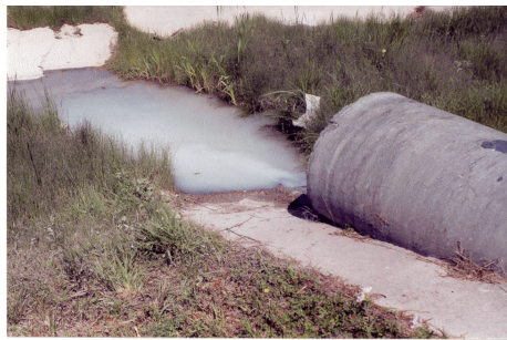
Figure 4. Source of white flow was grease from a fast food restaurant.
