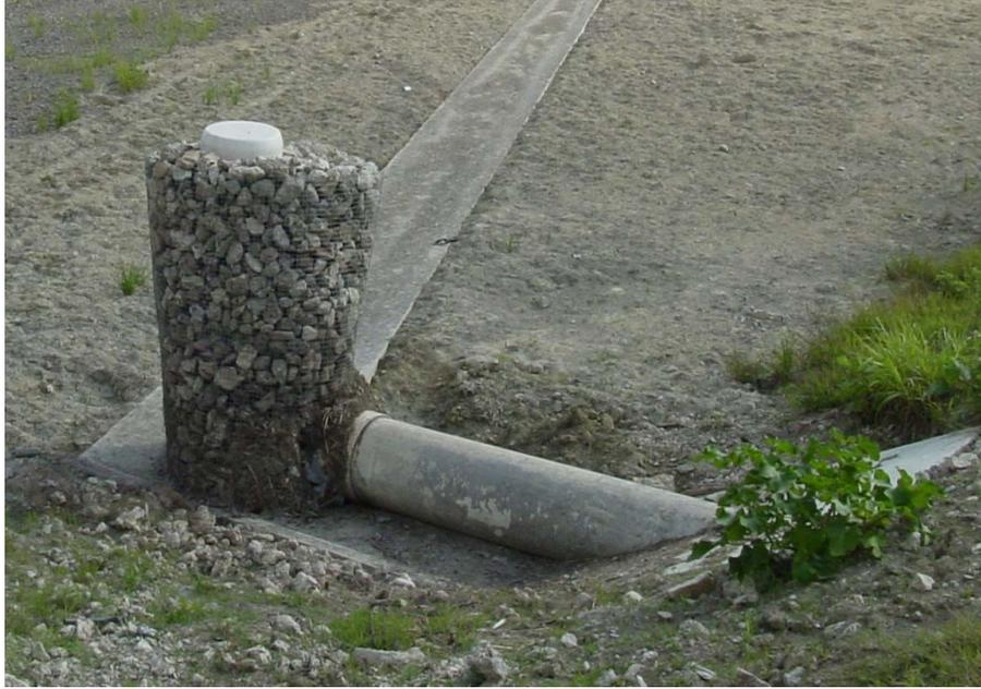
**Figure 4 Detail of Trash Rack**
