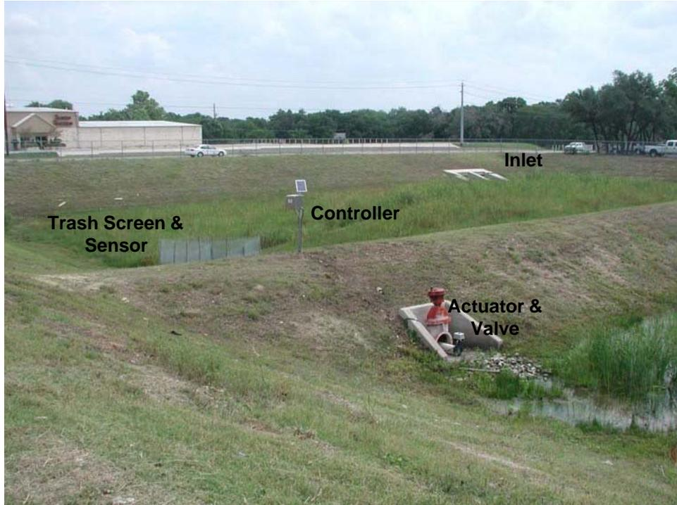
**Figure 2 Batch Extended Detention Basin**
