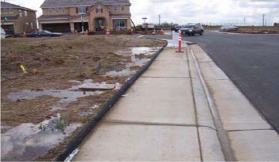
**Figure 1-44 SCR Installed Along a Sidewalk**
