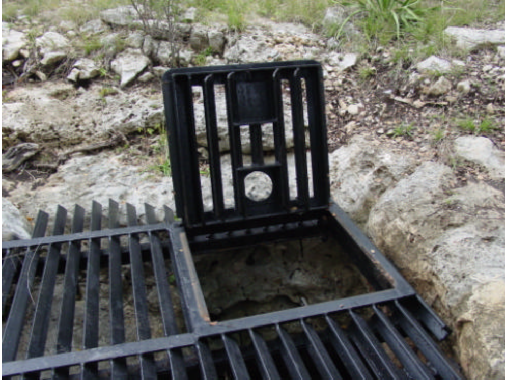
Figure 5-4 Example Cave Gate Access
