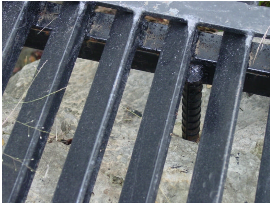
Figure 5-3 Example of Anchor Rebar
