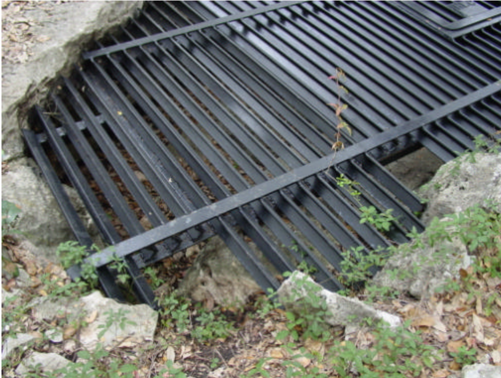
Figure 5-2 Mammal Access Portals Along Edge of Gate
