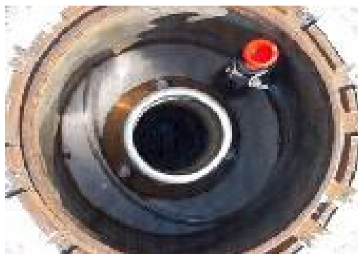
Figure 1. Spill bucket.
