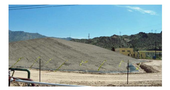
4. Looking at the third cell. The top of the waste material is approximately 14 feet above the ground which is over the design capacity.
