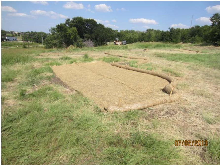
**Photo 12: Completed area with erosion mat and wattle.**
