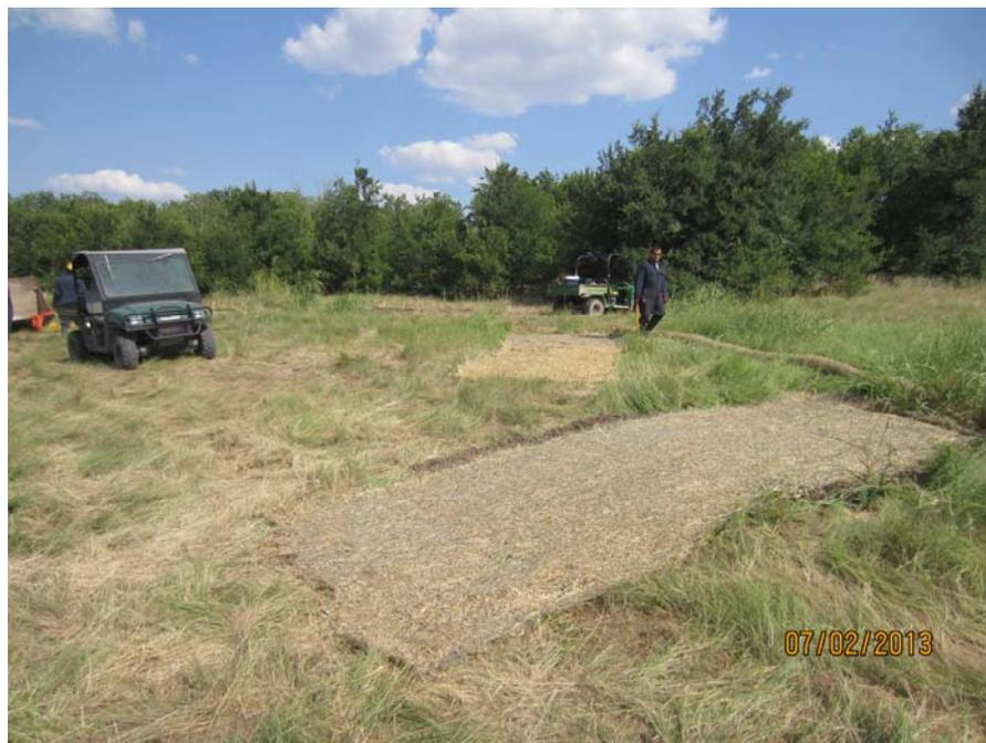
Photo 14: Completed area with erosion mat in place.
