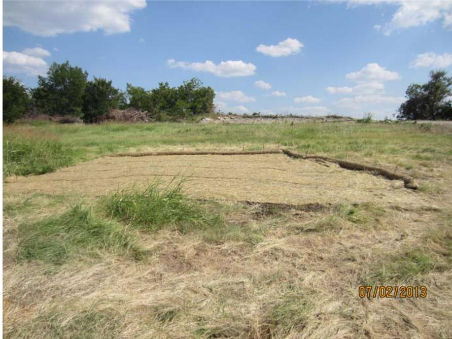
**Photo 11: View of repaired area after placement of seed and erosion mats.**
