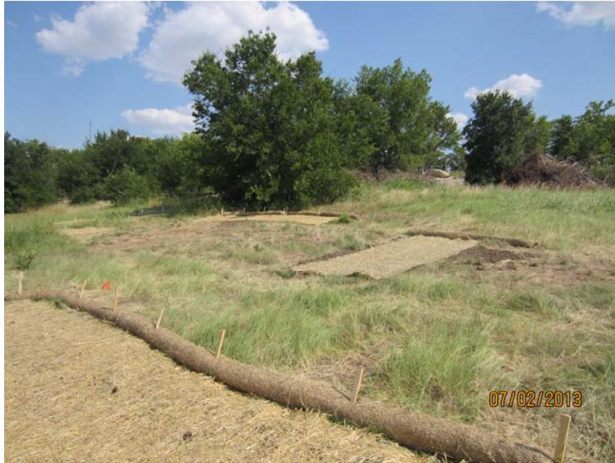
Photo 13: Multiple areas with erosion mat and straw wattles.
