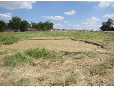
Photo 11: View of repaired area after placement of seed and erosion mats.
